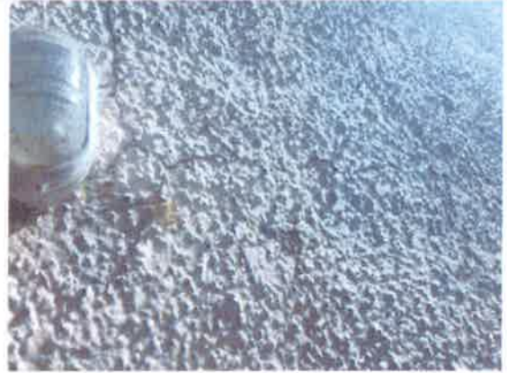
32 Gable Elevation – defective render adjacent to entrance door.
