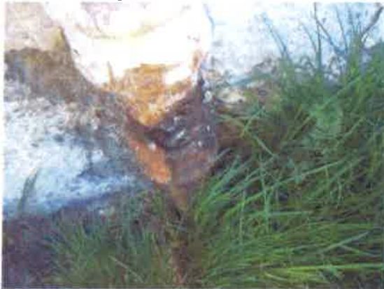
21 Defective cast iron downpipe at base.
