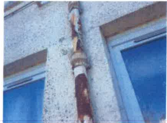
22 View of failed paintwork and heavy corrosion of cast iron downpipe.
