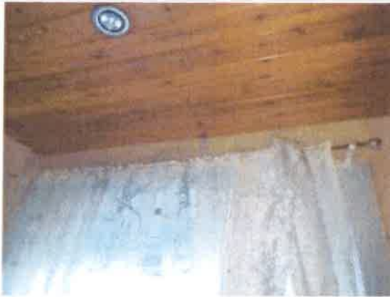
19 Area above kitchen window affected by high moisture readings.
