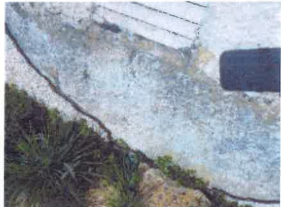
12 Close view of failure with overcoat render failing due to failure of bond.
