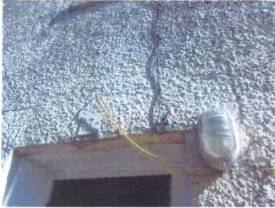
31 Gable Elevation – defective render adjacent to entrance door.
