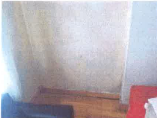
7 General view of recess adjacent to chimneybreast within Bedroom affected by dampness.
