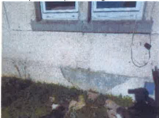
11 Area of defective render at basecourse over front elevation.
