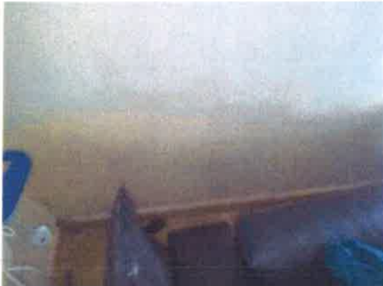
9 Low level to window wall within Bedroom – noticeably visual dampness staining.
