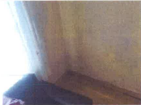
8 View of front corner – dampness at low level to window wall and extending to recess adjacent to chimneybreast.
