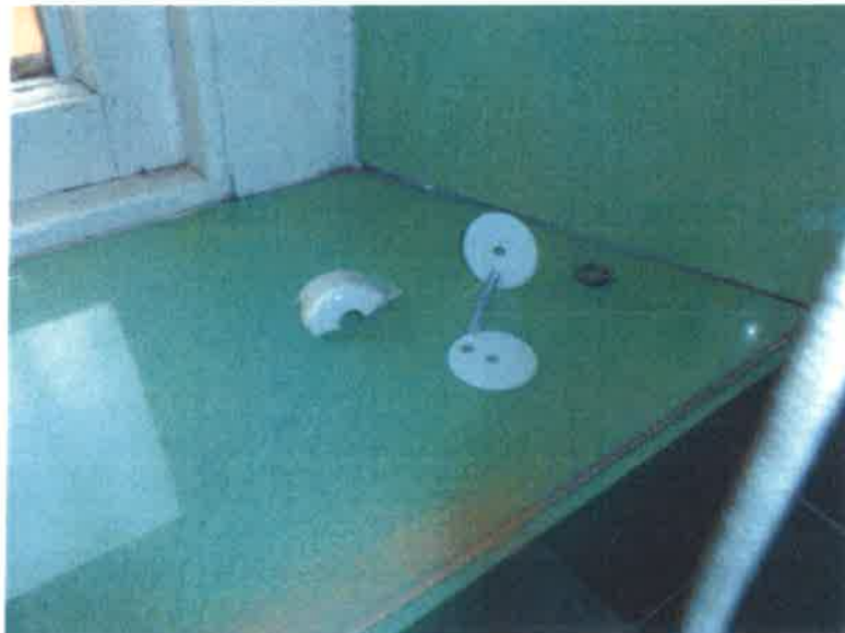
8. Broken section of WC pedestal
