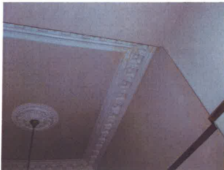
11. Water damage to ceiling/cornice in hall
