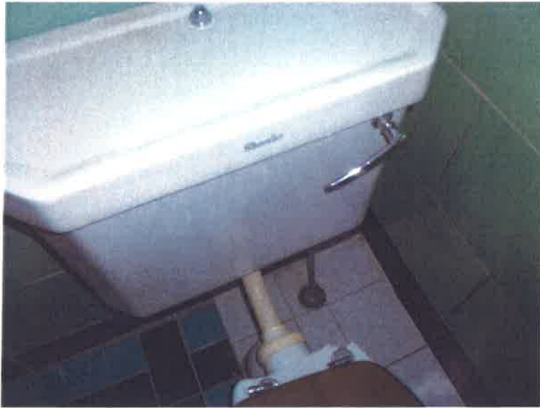
7. WC cistern– not flushing
