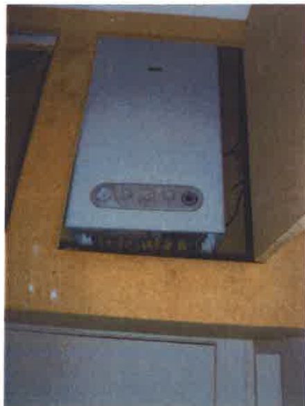
2. Gas central heating boiler
