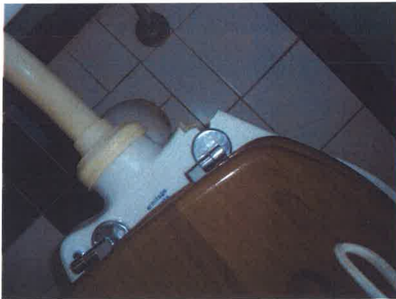
6. WC pedestal – broken at seat fixing
