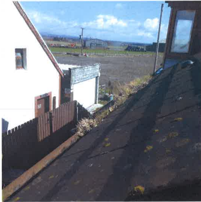
5 Example of weed build up in the gutters to the rear
