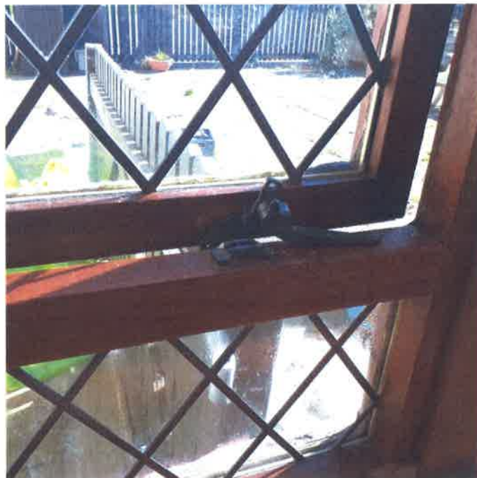
6 Example of defective window ironmongery
