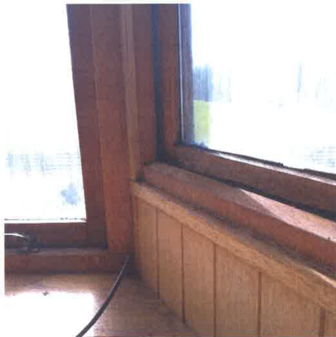
8 Example of ill-fitting window unit (first floor front bedroom)
