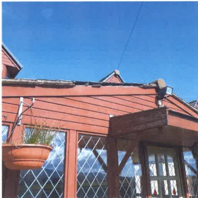
4 Missing/displaced mortar fillets at front elevation sun room porch
