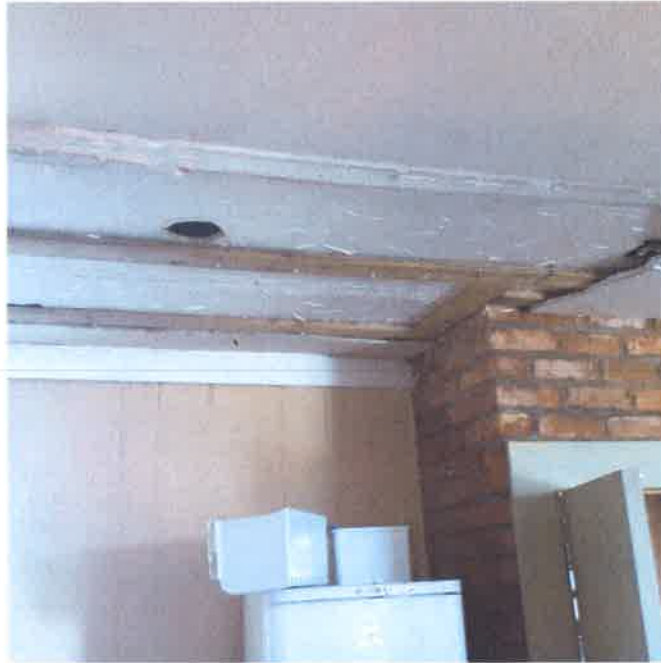
9 Part collapsed ground floor kitchen ceiling; water staining noted on wall
