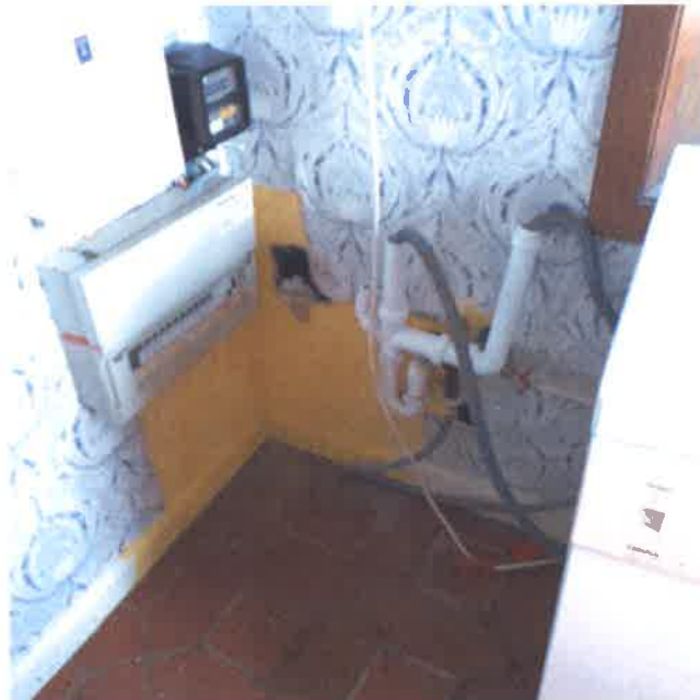
12 Electrical switchgear and ad-hoc washing machine plumbing in ground floor utility room
