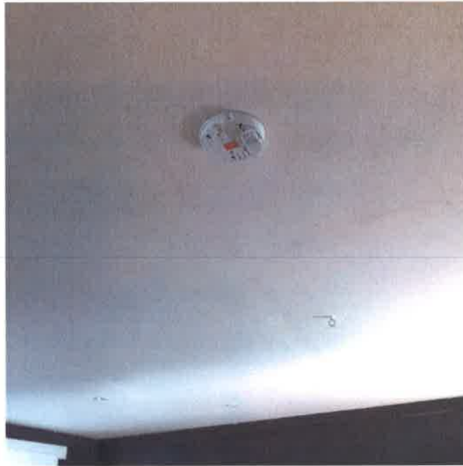
13 Defective ceiling mounted smoke detector in ground floor kitchen
