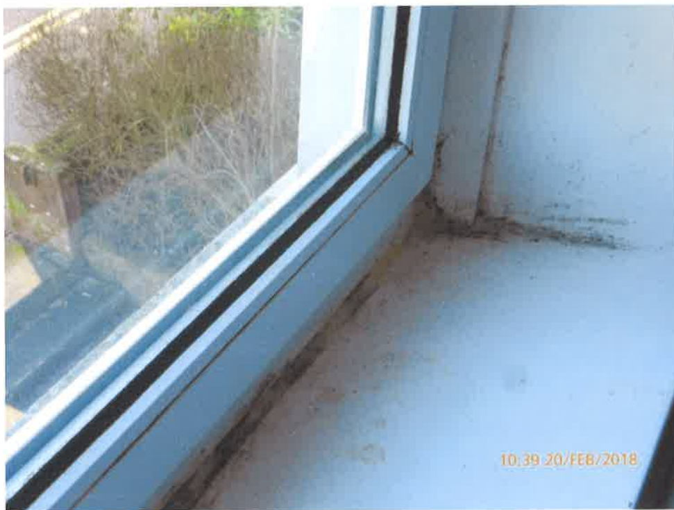
Condensation mould
