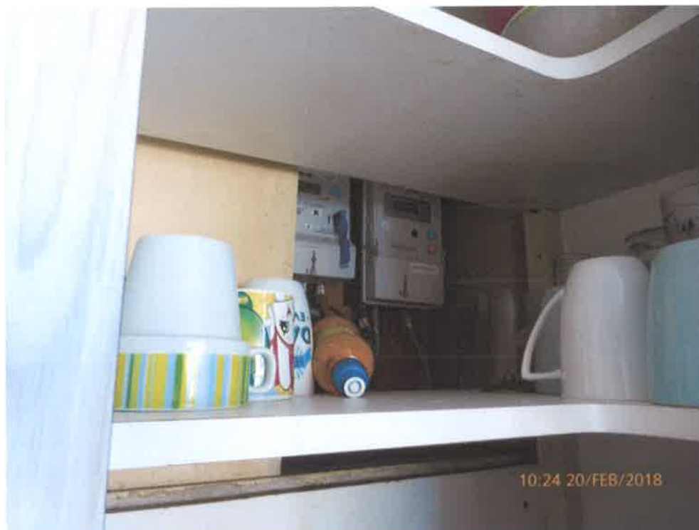
Electricity meter behind a kitchen cupboard
