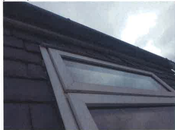
32 Poor detailing of slate above kitchen window.
