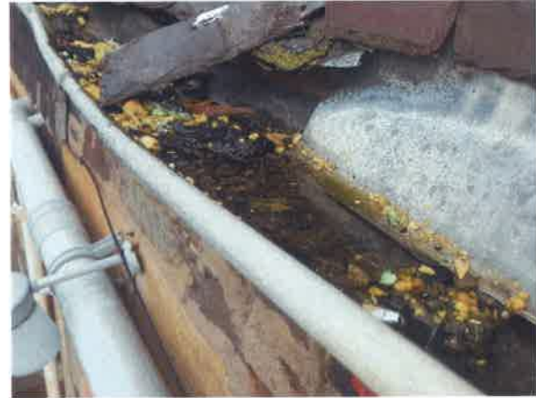
26 Undulations and deformation to defective lead gutter.
