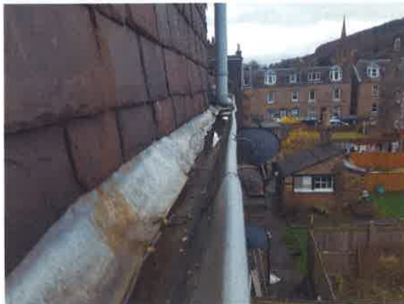
25 Lead gutter to rear roof pitch.
