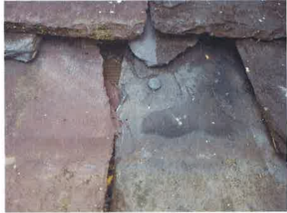
30 Exposed sarking to tiles (no underslating felt present)
