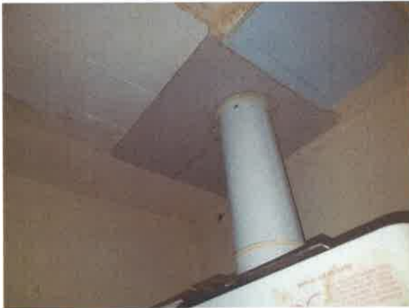
23 Boiler flue and access hatch.
