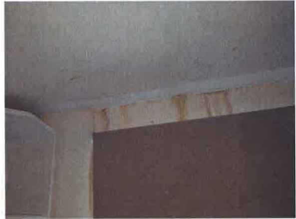
14 View within Kitchen above window of water ingress damage.
