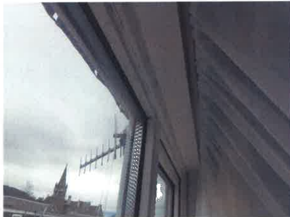
9 View to head window frame and isolated staining from water ingress.
