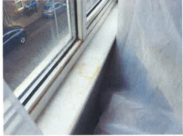
8 View within Living Room tripartite window – staining at sill.
