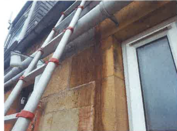
34 Water escape staining from defective gutter.
