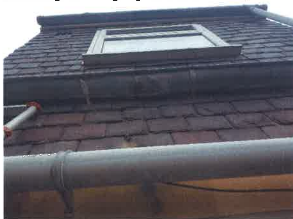
33 Defective joint to lead gutter.
