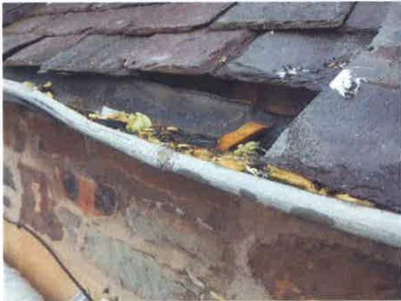
29 Close view of deformation and ponding water within gutter.
