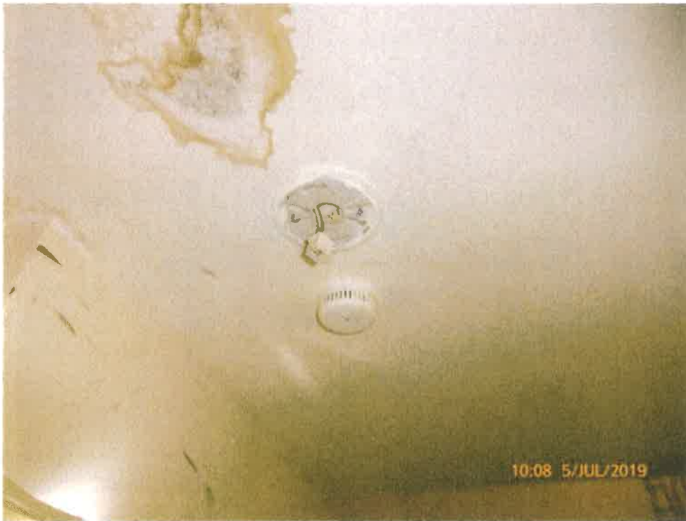
Hard wired smoke detector removed
