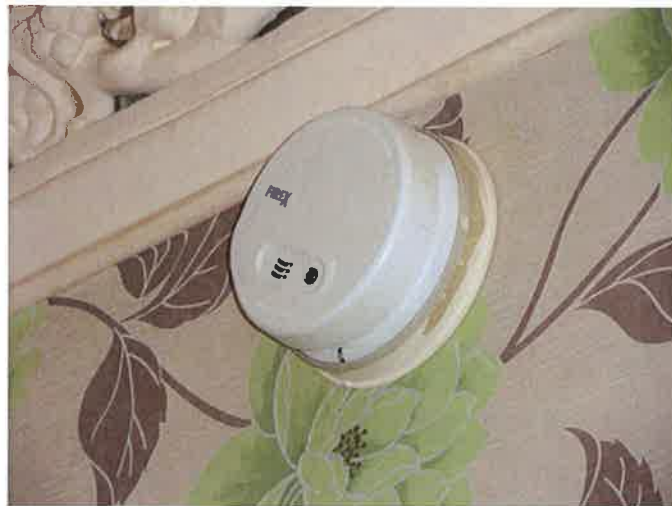
Photograph 4: Wall mounted, hard wired smoke detector in living room
