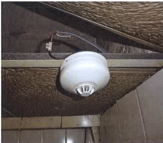
Photograph 2: Ceiling mounted hard wired heat detector kitchen
