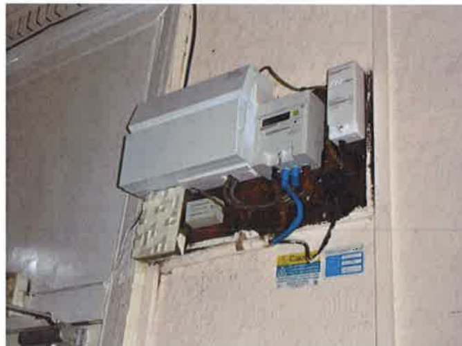
Photograph 5: Electrical consumer unit wall mounted in hall
