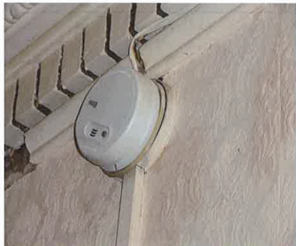
Photograph 3: Wall mounted hard wired smoke detector in hall.
