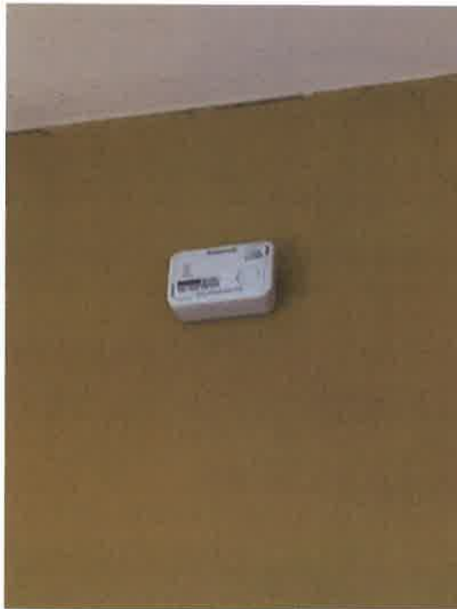
Photograph 15: carbon monoxide detector
