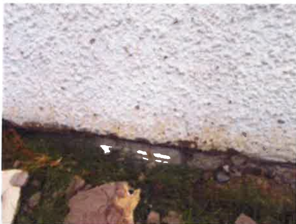
External - Front elevation - underfloor vent below ground level
