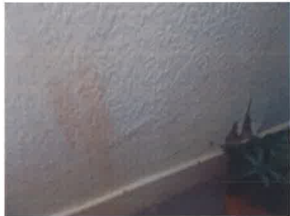
Bedroom (4) - UF to front - water stain and damage to wallpaper under window
