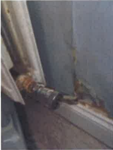
Kitchen - Thermostatic control valve to radiator part missing
