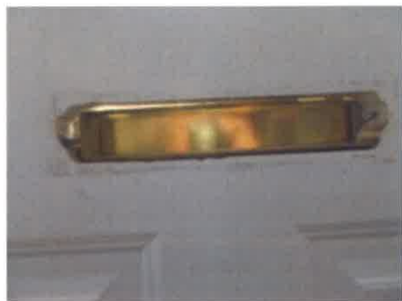
Hall - Front door - missing flap to letter box - internal view
