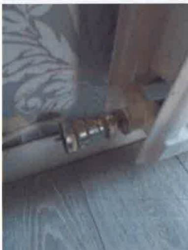
Hall - Ground Floor - Thermostatic control valve to radiator - part missing
