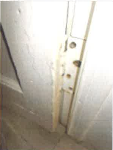
Bedroom (1) - GF to front - Door hinge to base defective/missing/broken screws
