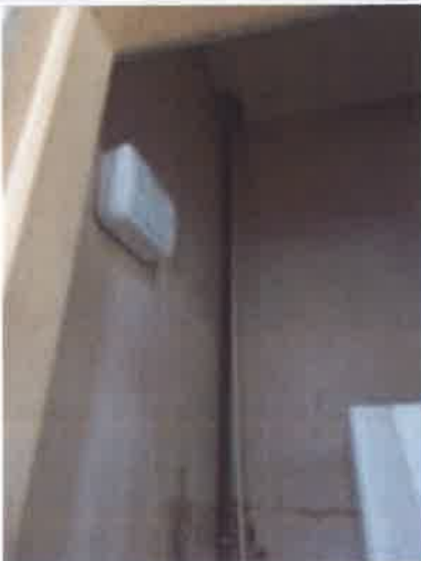
Bedroom (3) UF to rear - CO alarm wall mounted within boiler cupboard
