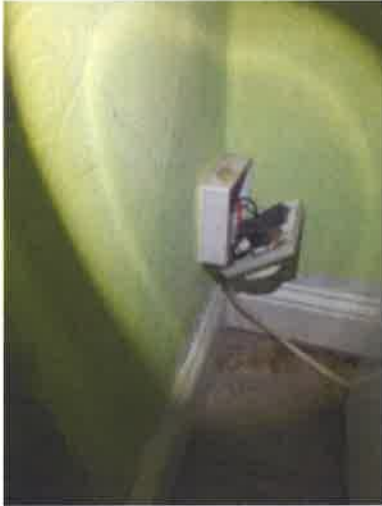
Kitchen - single socket cover loose/wires exposed
