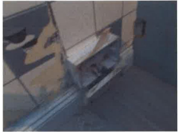
Kitchen - double socket cover loose/wires exposed
