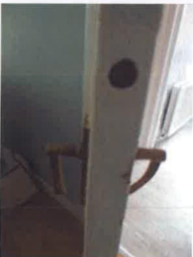
Living Room - Defective door handles, missing ball catch
