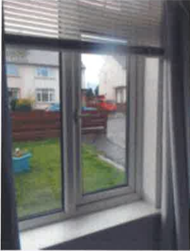
Bedroom (1) - GF to front - window does not open, handle defective/loose
