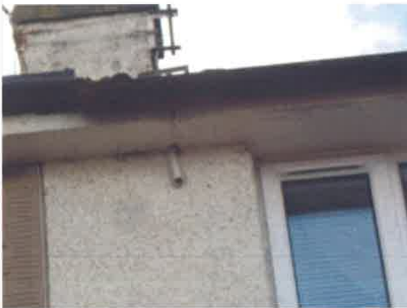
Rear external elevation - gutter defective/leaking at joints and choked with vegetation
