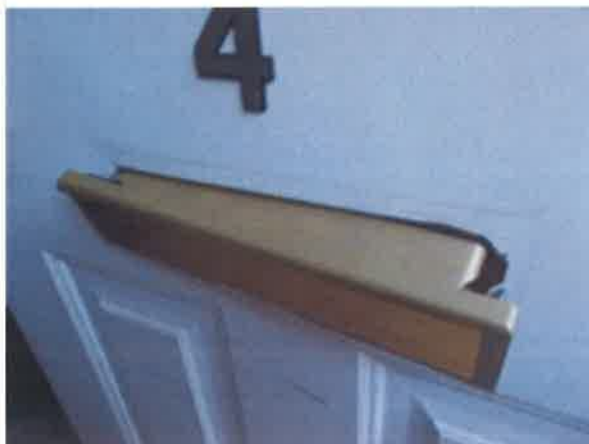
Hall - Front door - letter box defective/ not secure - external view
