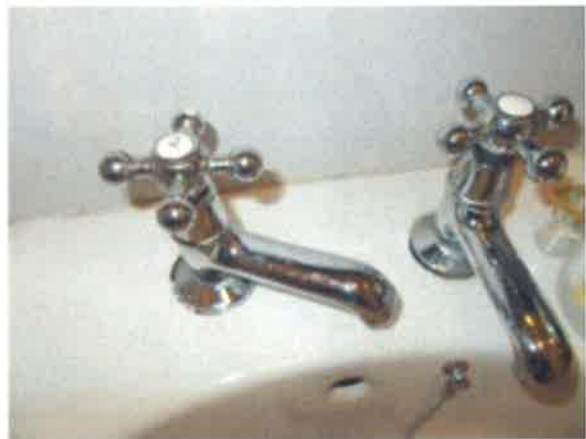
Ground floor toilet - Hot water tap not fixed properly/defective/no hot water
