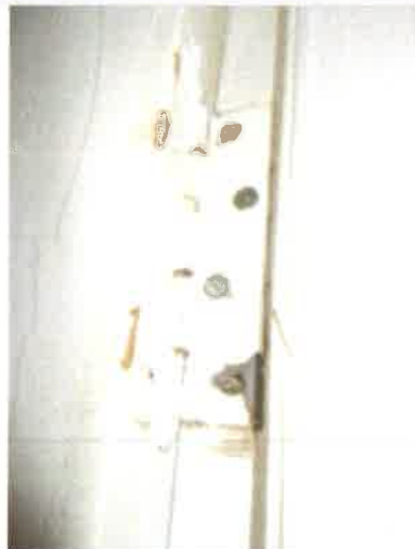
Bedroom (1) - GF to front - Door hinge at top defective/missing/broken screws
