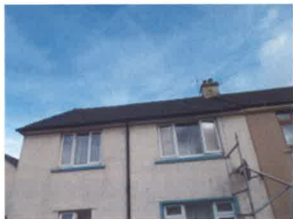
Front external elevation - gutter defective/leaking at joints and choked with vegetation
