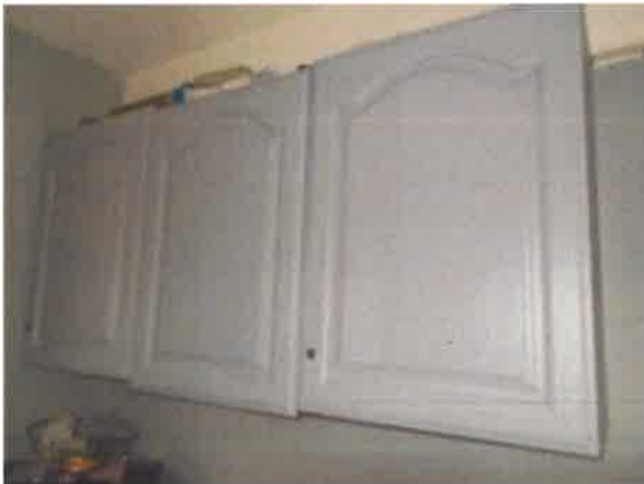
Kitchen - Wall mounted units misaligned and several handles missing
