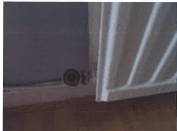
Living Room - Thermostatic control valve to radiator part missing
