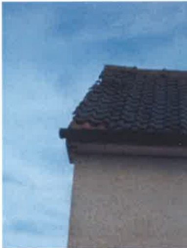
Front roof pitch - loose roof tiles at verge (Observation)
