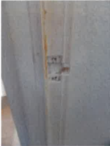
Bedroom (4) - UF to front - Door - ball catch plate at jamb missing
