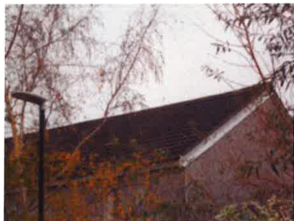
Front pitch of roof
