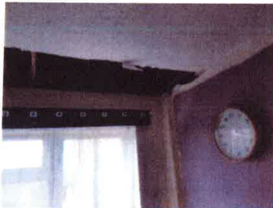
5 View of collapsed ceiling.
