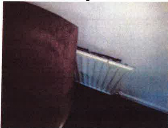
15 Central heating pressed panel radiator.
