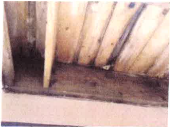
2 Water staining to underside of Bathroom flooring.
