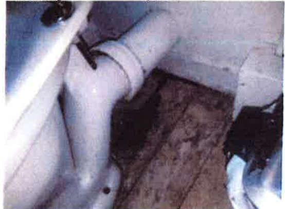
24 Water staining below WC waste.
