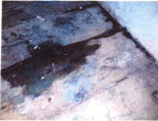
25 Close view of water stain below WC waste.
