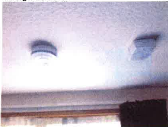
9 Smoke detector and CO alarm within Living Room.
