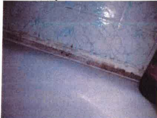
35 Incomplete wall tiling to bath.
