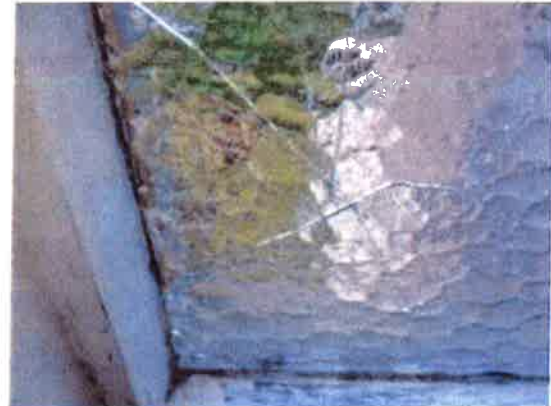
36 Cracked glazing.
