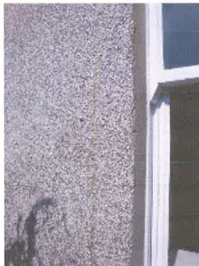
9. SILICONE SEAL AT RENDER CRACK.
