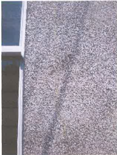
10. SILICONE SEAL AT RENDER CRACK
