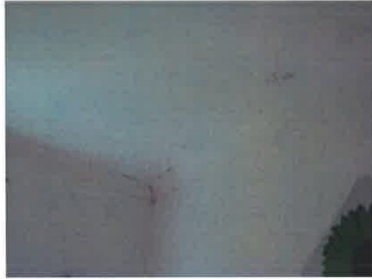
MAIN BATHROOM-WINDOW SEALED AND CONDENSATION STAINS ON CEIL.
