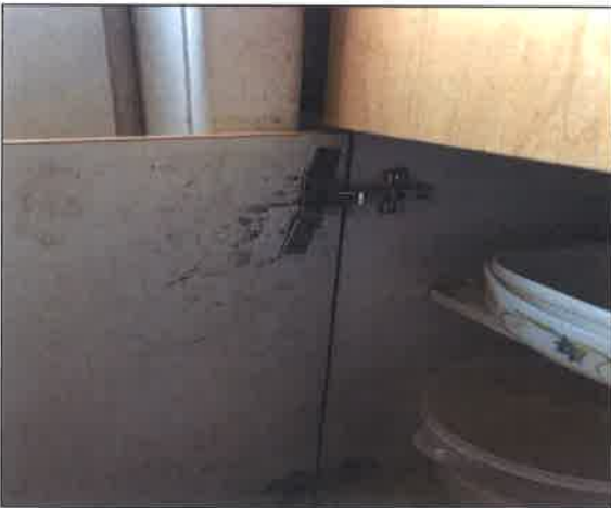
The repair to the cupboard hinges are not to a reasonable standard and the protruding screws could be dangerous
