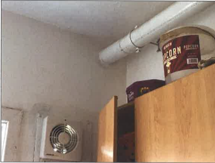
Hole at gas boiler flue repaired.
