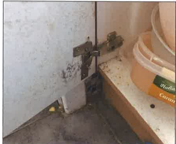
The repair to the cupboard hinges are not to a reasonable standard and the protruding screws could be dangerous
