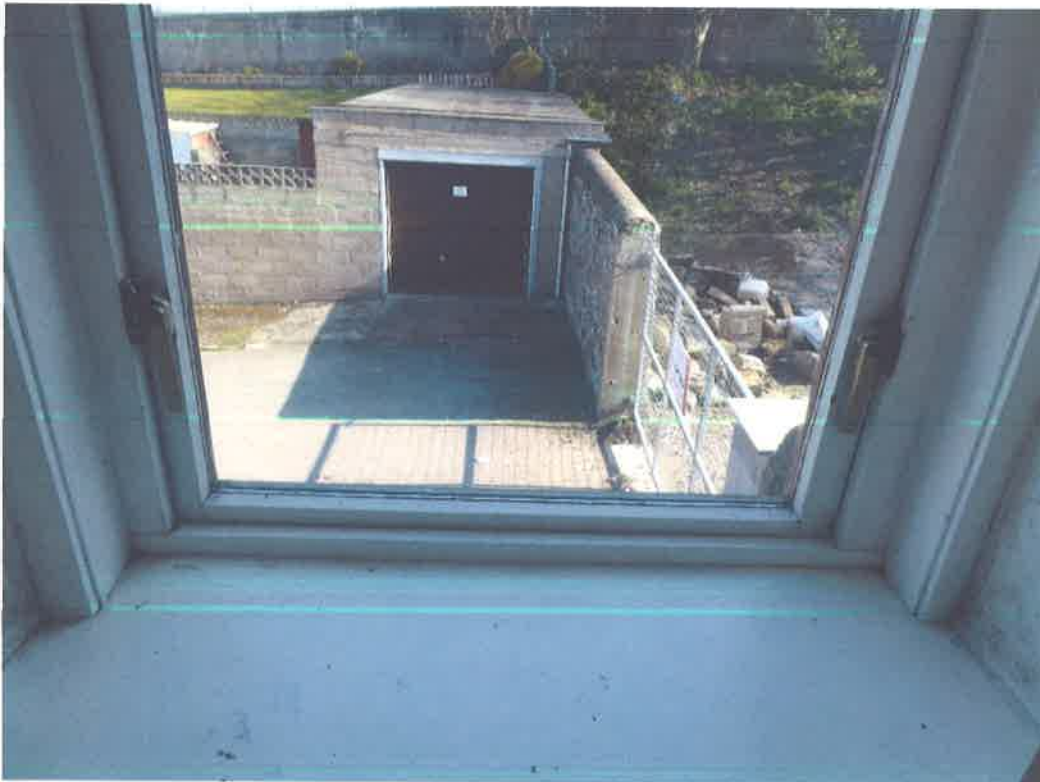
1 st floor bedroom right – both catches in working condition
