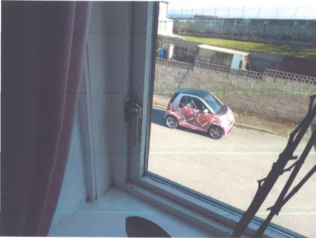
1 st floor bedroom left – catch in working condition (other catch also in working condition)
