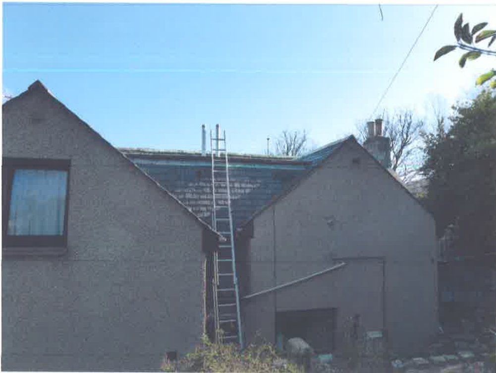
Rear elevation (1 & 2 share a flat roof) 1 is to the right.
