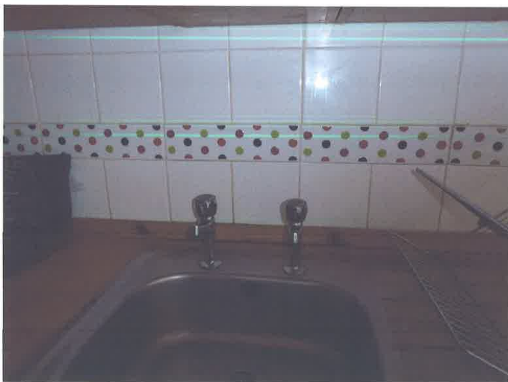
Kitchen sink. Dripping / loose hot tap has been repaired.
