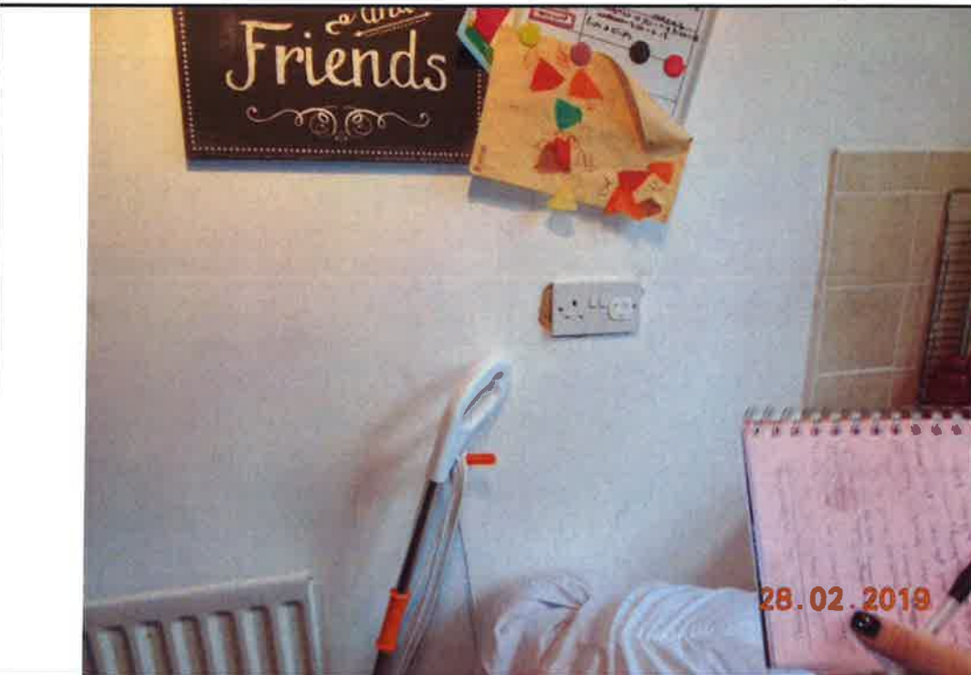
24. Hole in plasterwork around electrical socket outlet in Kitchen
