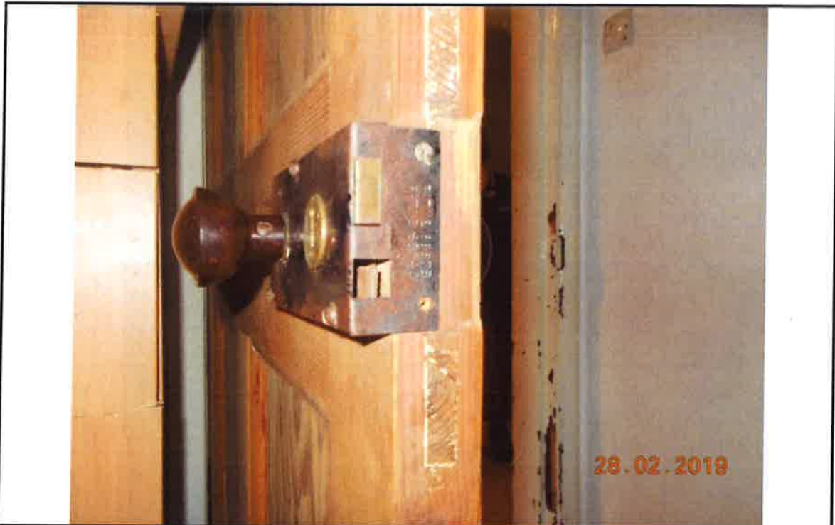
27. Door lock with missing catch in other Front Bedroom (typical)
