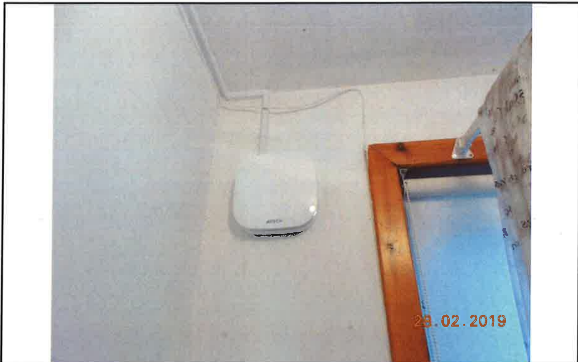
15. New extract fan fitted in Bathroom
