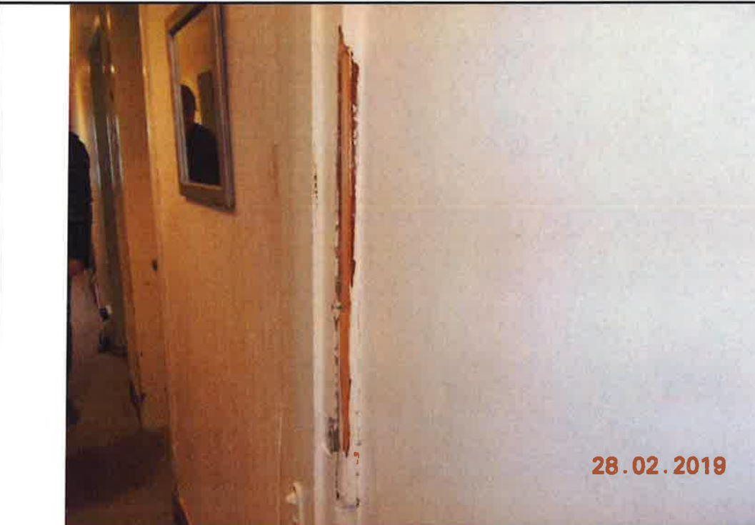
30. Damaged timber surround to door to Bathroom
