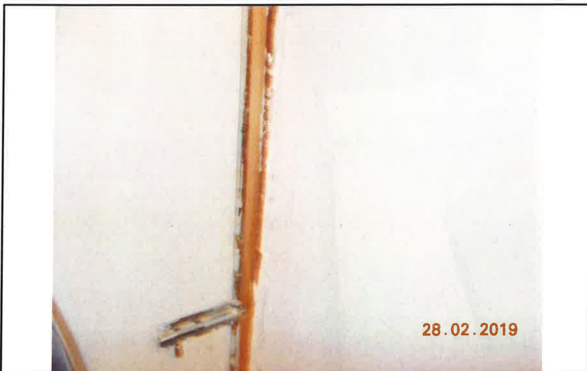
31. Damaged timber surround to door to Bathroom
