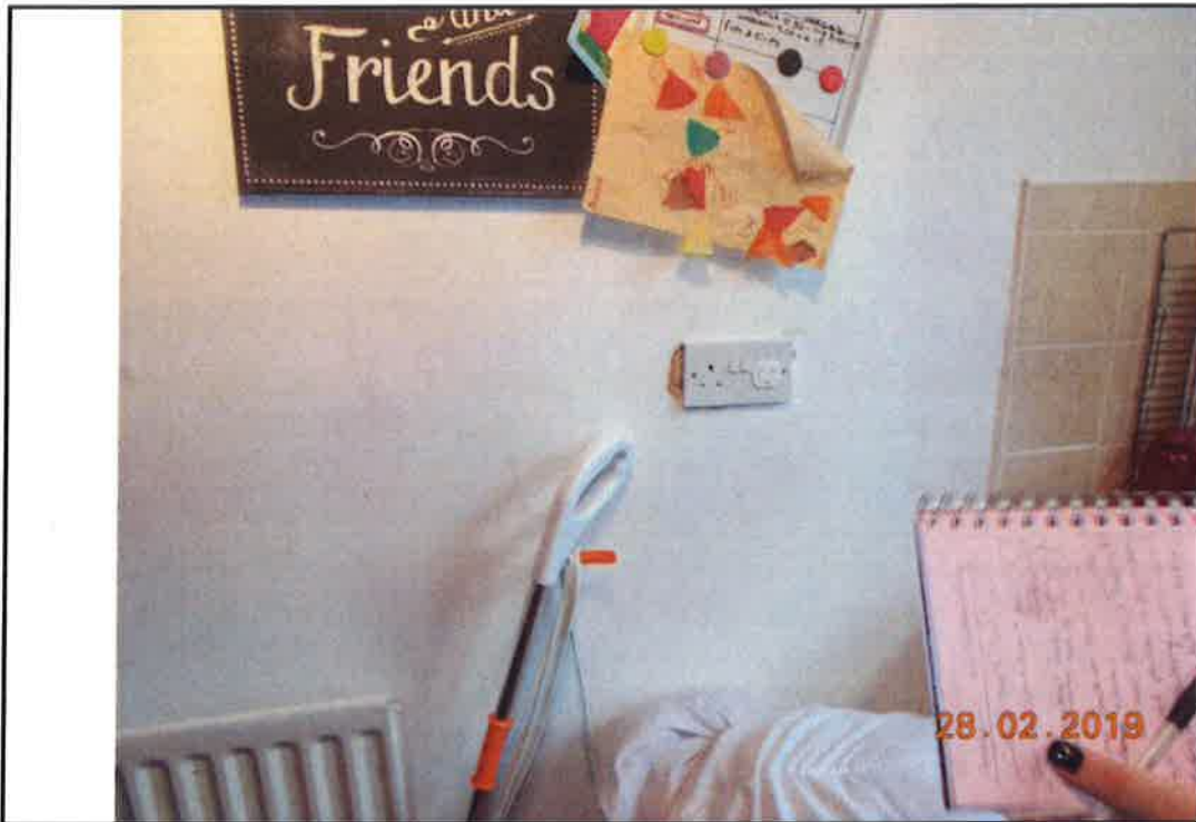
37. Gap at side of electrical socket outlet in Kitchen
