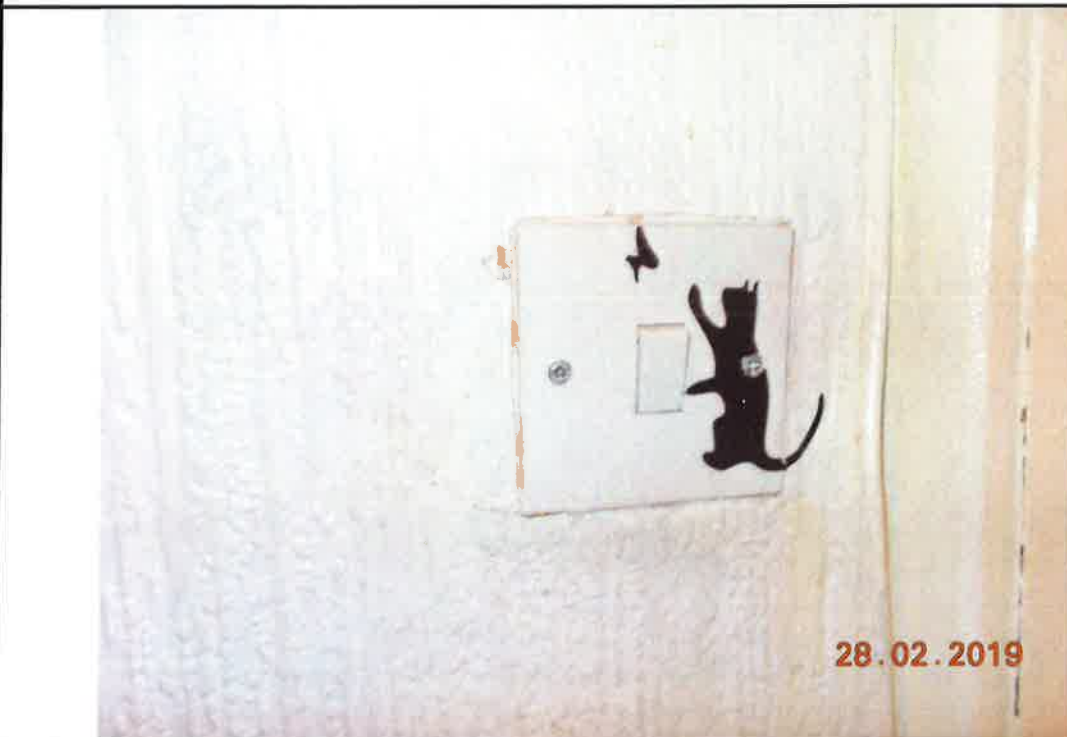
38. Loose light switch in Hall serving Bathroom light
