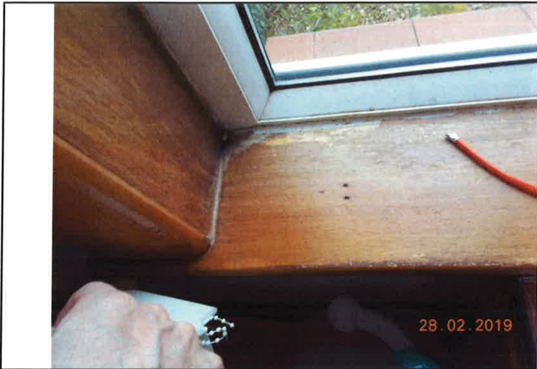
13. Damp/mould at window in Living Room
