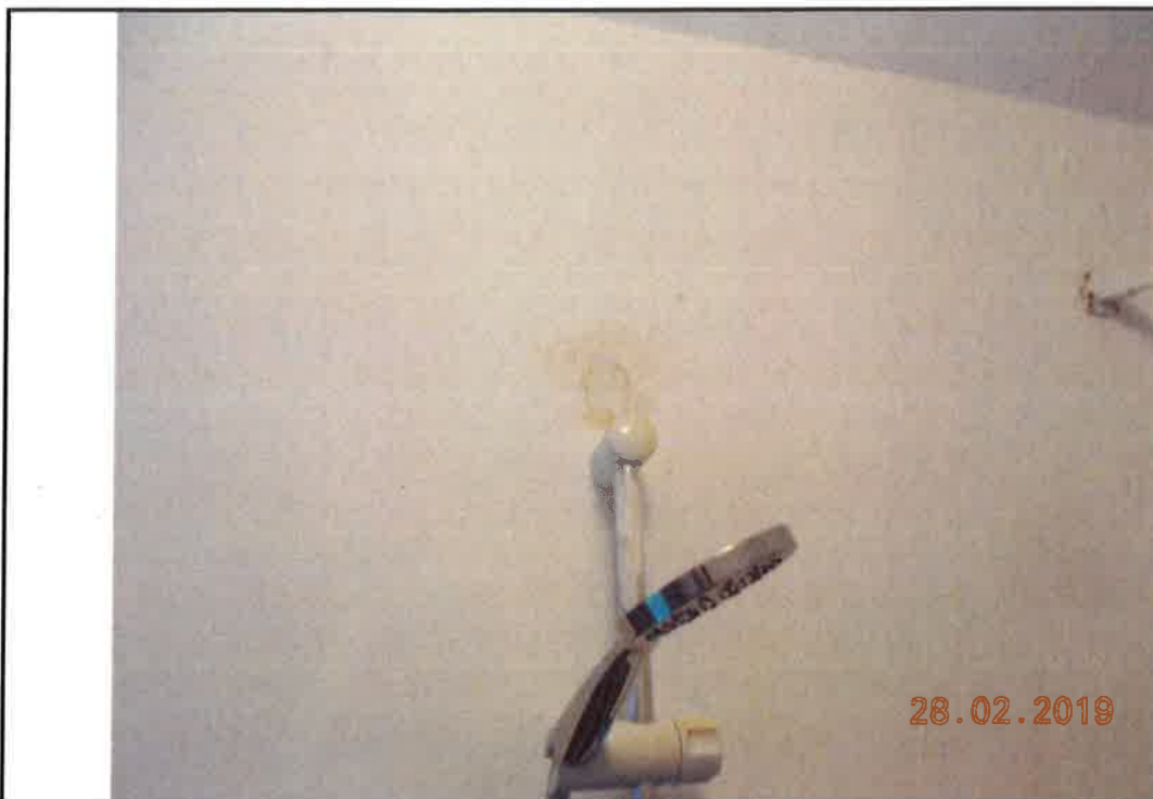
9. Patched plaster/decor at shower fixing in Bathroom
