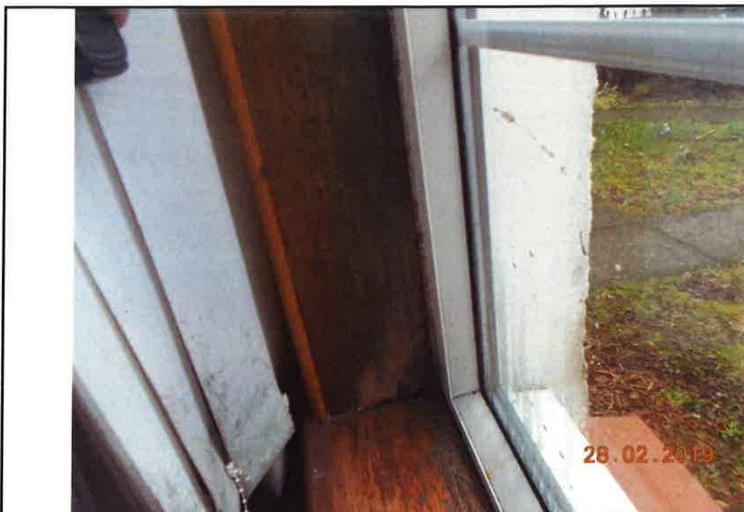
11. Damp/mould at window in main Front Bedroom (left on entering)
