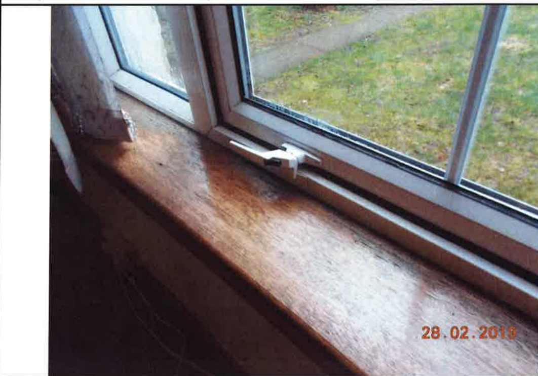
10. Damp/mould at window in main Front Bedroom (left on entering)
