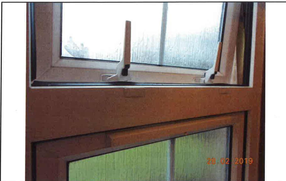
21. Seal to opening section of window in Bathroom
