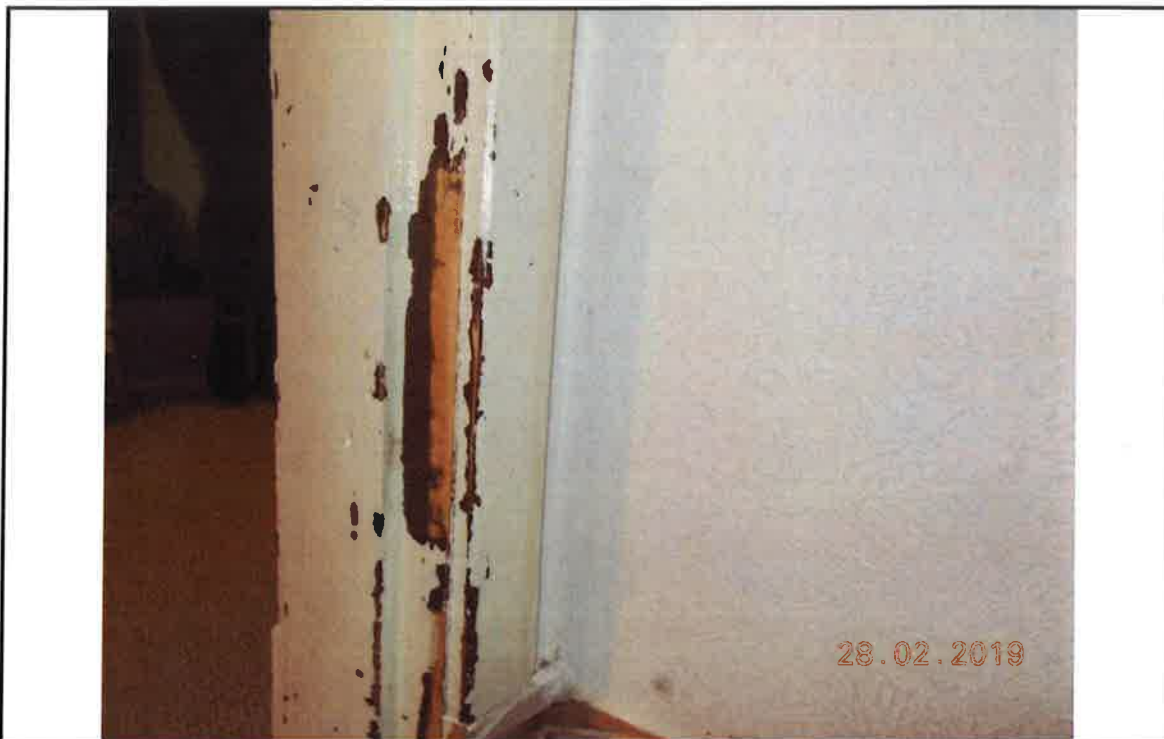
5. Decor damage to door surround in second Front Bedroom (right on entering)
