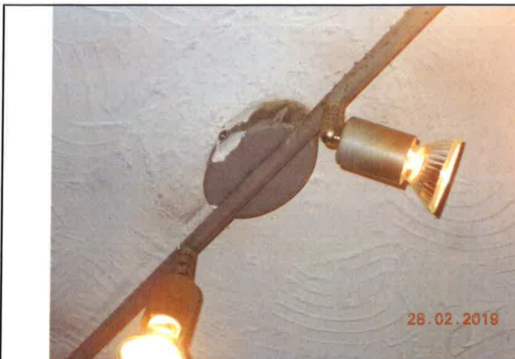
41. Loose light fitting in Kitchen
