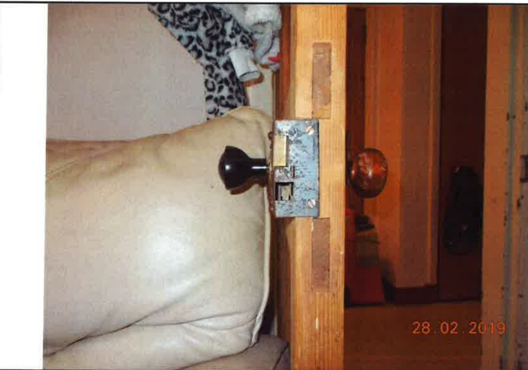
28. Door lock with missing catch in Living Room (typical)
