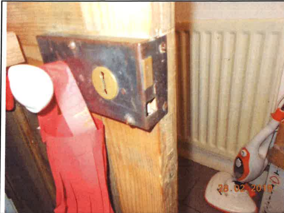
29. Door lock with missing catch in other Kitchen (typical)
