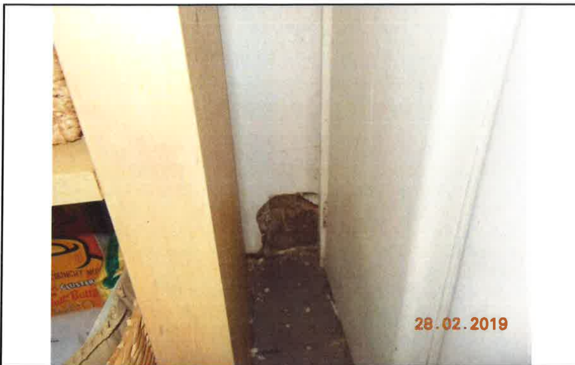
25. Hole in plaster work on inner surface of gable wall in Kitchen
