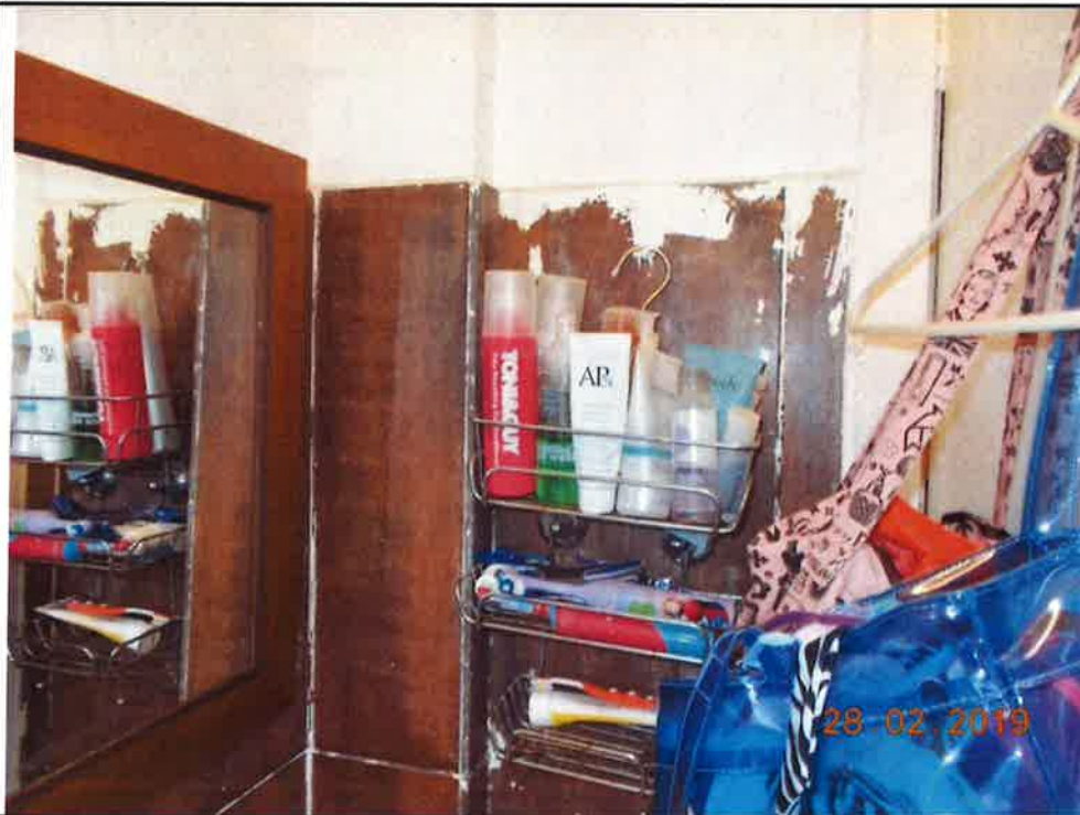
8. Stripped decor from tiles in Bathroom
