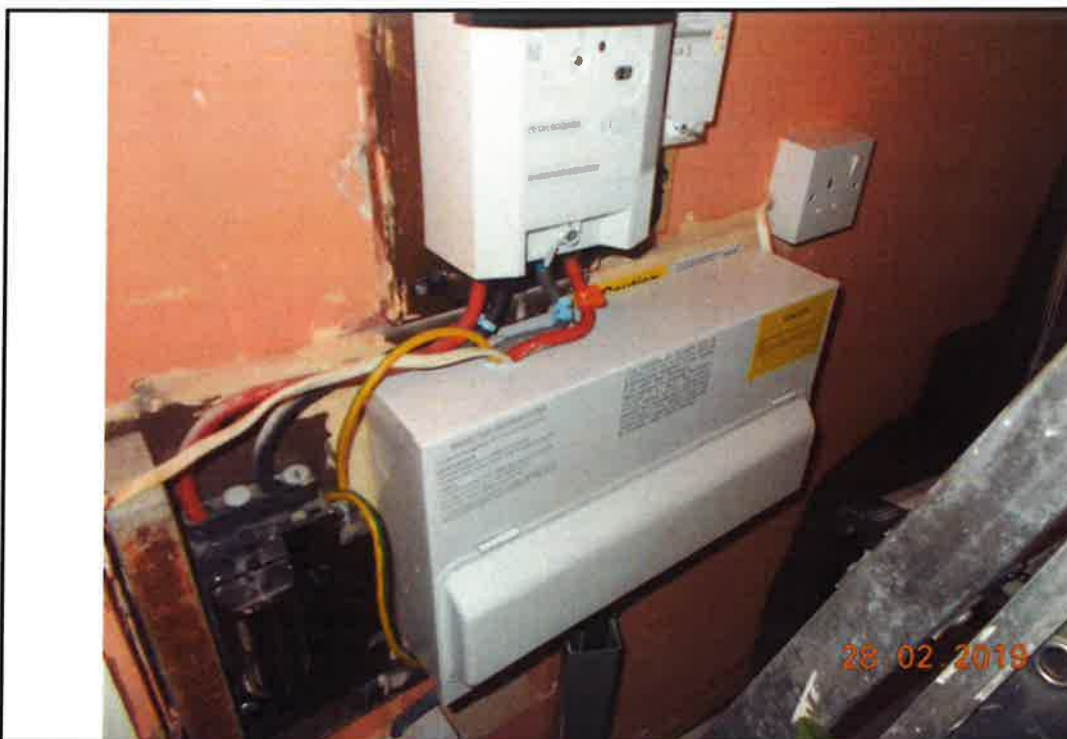
39. Consumer Control Unit for electrics in cupboard off Hall
