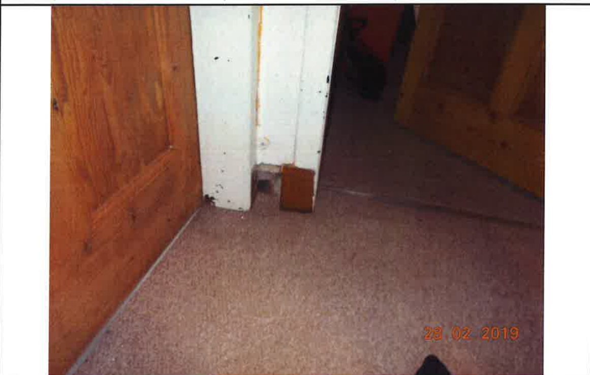
22. Missing section of skirting board in Hall (hole in wall)
