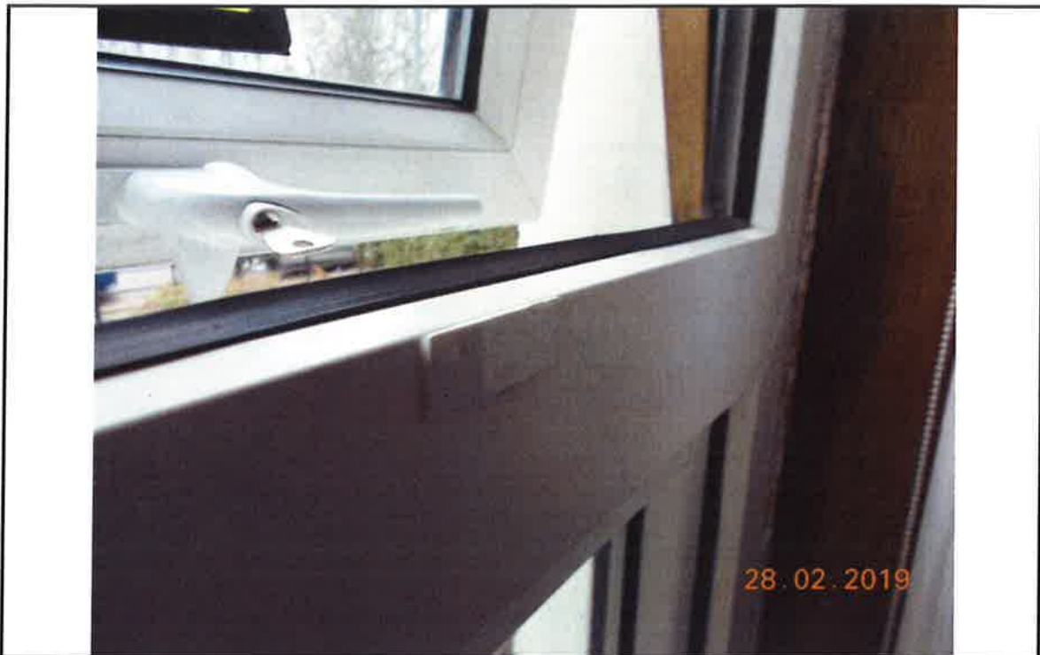
17. Seal to opening section of window in other Front Bedroom (right on entering)
