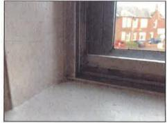
Single glazed window with a secondary glazed unit fitted. The secondary glazing unit is damaged at both corners due to a sudden drop and sits twisted within the frame. Parts of window frame have been taped over.
