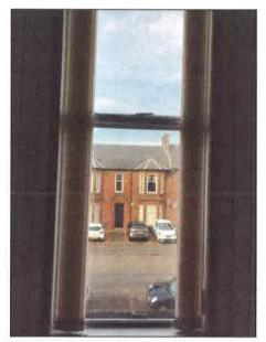
Single glazed window with a secondary glazed unit fitted. The secondary glazing unit is now twisted within the frame and is no longer secure.
