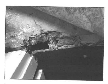
Rotted floor timbers at bathroom door - vinyl floor covering lifted
