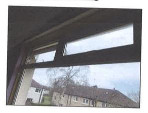
Windows tested only one hopper opens, no key to lock. No evidence of dampness Condensation noted within window panel - Appears seal has failed
