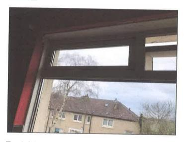
Top left hopper unable to open - possibly locked - No key to check. No evidence of dampness
