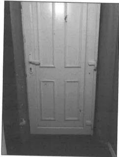
Upvc facings are missing internally and door is not wind and water tight
