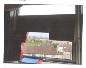
The only escape window within the property appears to be propped up/wedged with cardboard, Unable to open as window unit may fall out.
