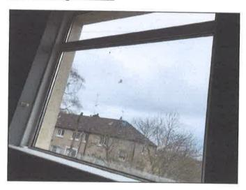
Fixed pane. Mould visible due to condensation
