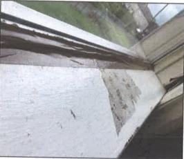
Lounge window - Top left hopper and window unit taped closed, a cable appears to be running from outside and the handle is broken. Window sill and surrounding areas tested for dampness all readings within normal range
