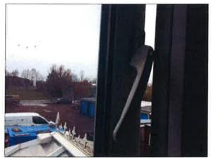
Window handles in front bedroom back bedrooms are broken and fail to lock. The windows are no longer wind and watertight and fail to secure the property.
