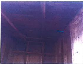
Outhouse roof appears to have been constructed with timber with a felt covering. The timber has rotted and the felt has been replaced with a tarpaulin. The structure is no longer water tight.
