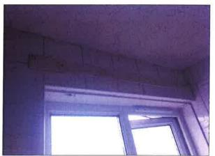
Evidence of condensation/mould is visible within the bathroom. I would advise that adequate heating and ventilation is required to address this matter.
