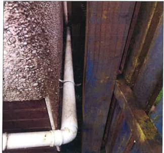
Rain water pipe at the rear extension is disconnected at the existing downpipe rain water is discharging into neighbouring garden
