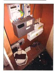
A new consumer unit has been fitted along with an isolating switch.
