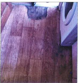
Water damage to kitchen ceiling and vinyl flooring from the upstairs bathroom due to a previous repair by the property factors contractor.
