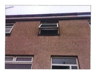
Render at the front door, lounge and bedroom window is loose, missing and brickwork is visible.
