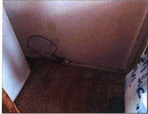
No radiator has been fitted within the kitchen, however, the pipe work and TRV is in situ and forms part of the central heating system causing a potential hazard
