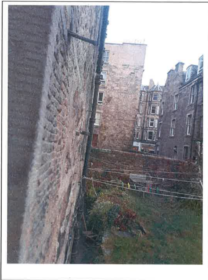
View from kitchen window showing rear elevation with external gas vent
