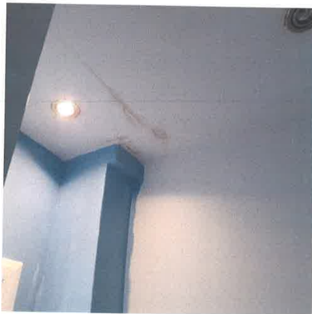
4 The damaged ceiling at ground floor level below the bath
