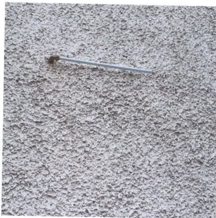
7 The redirected boiler overflow on the front elevation
