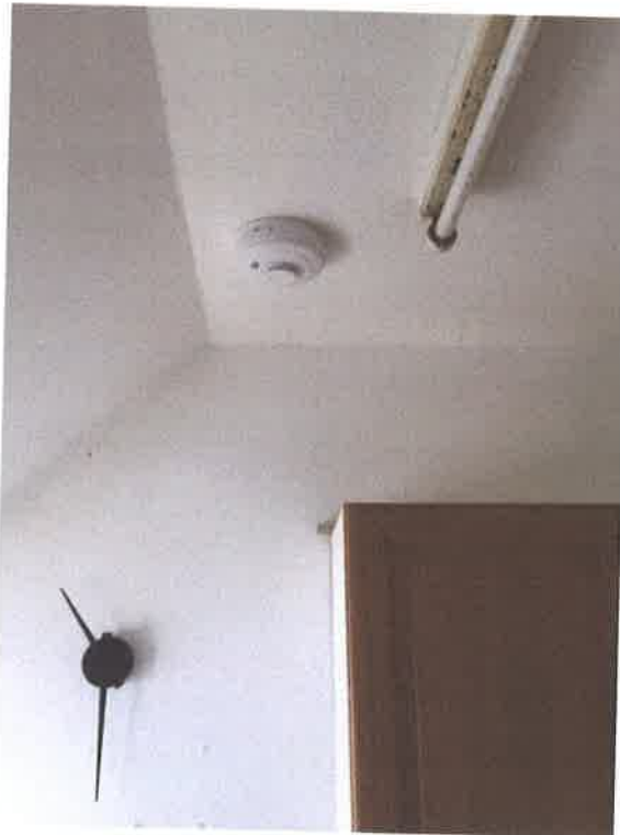
Photograph 7: Kitchen: heat detector
