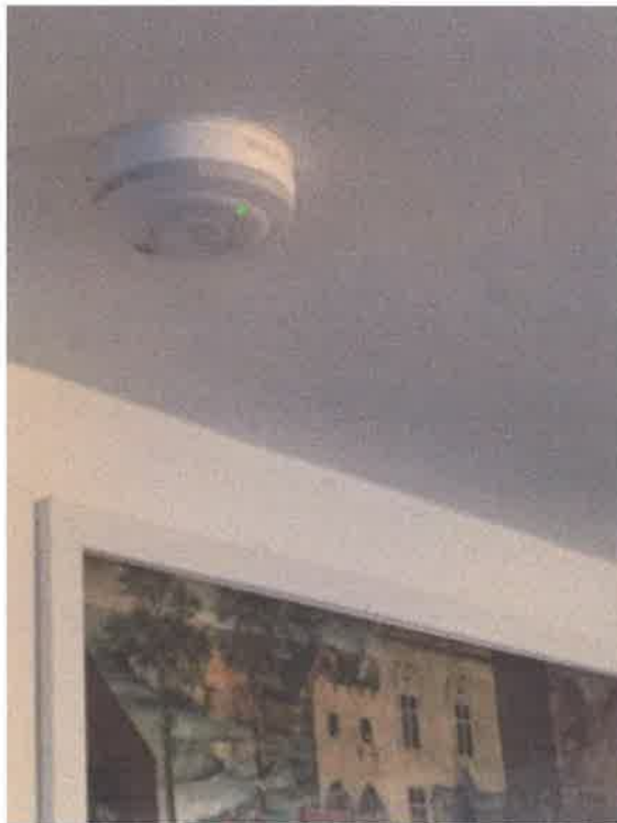
Photograph 9: Living room: smoke detector
