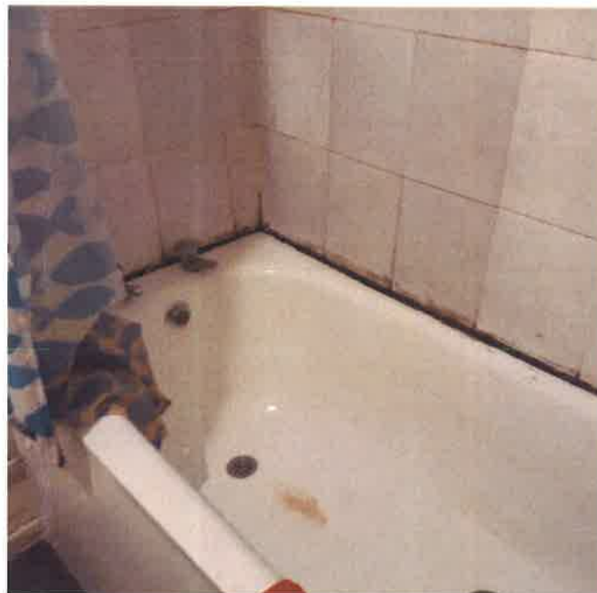
4 The mould on the bathroom tiling
