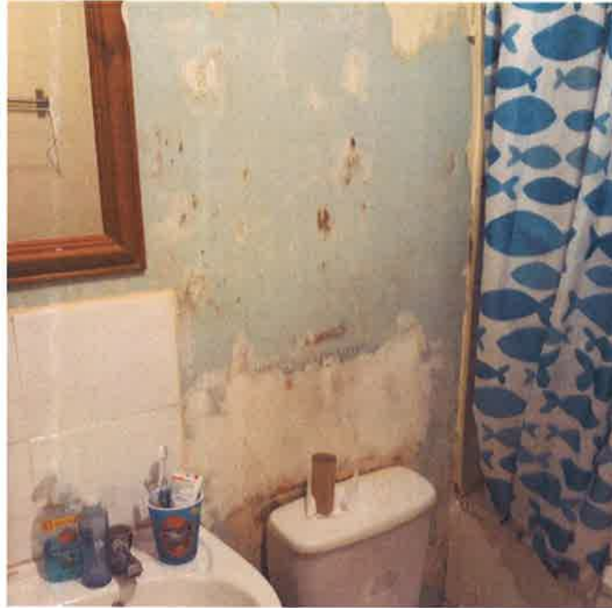
3 The mould on the bathroom walls
