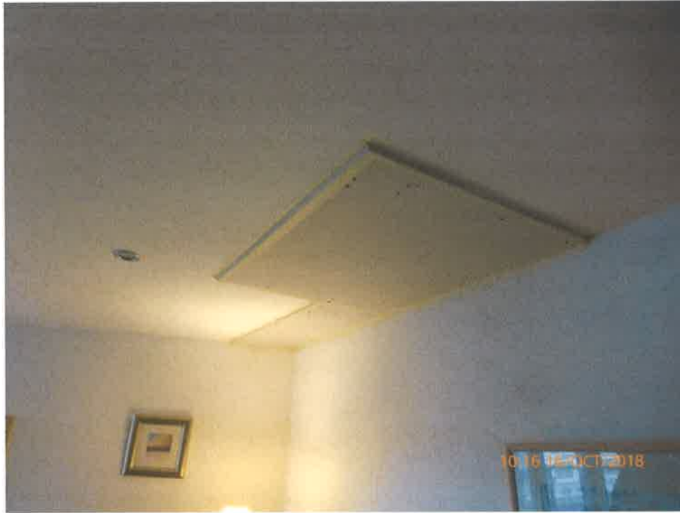
Other areas of ceiling cut for inspection
