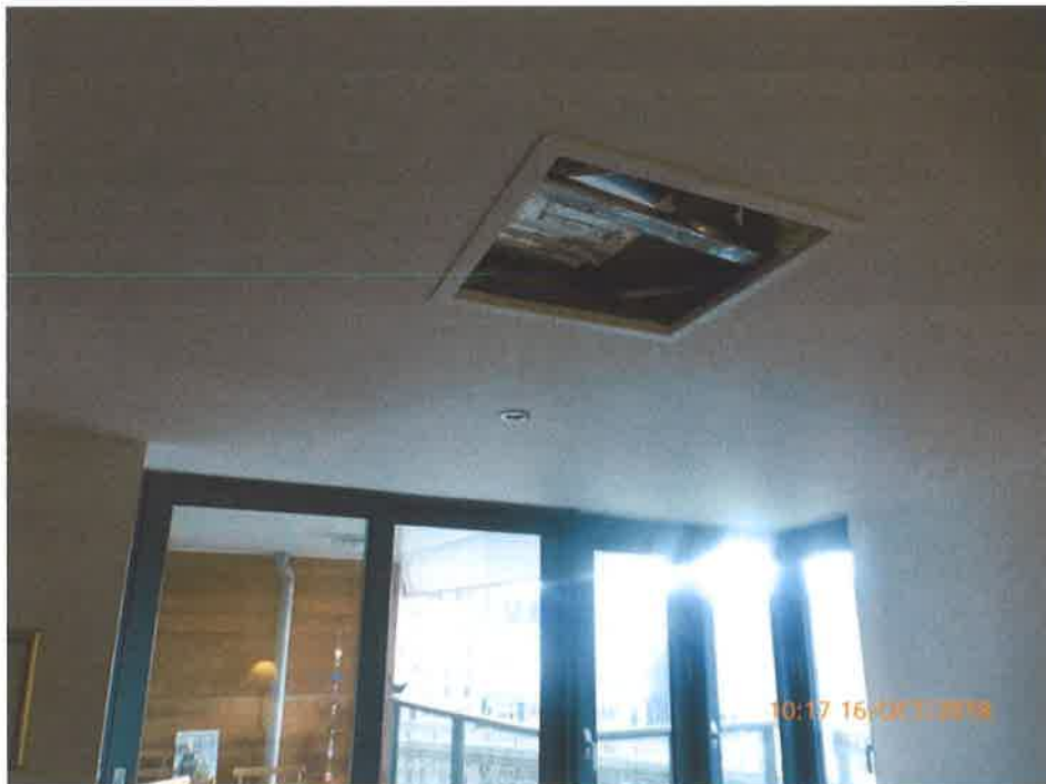
Hatch cut in ceiling
