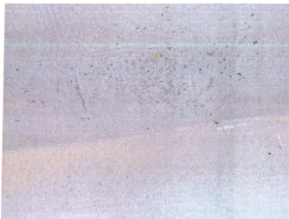
18. Condensation on Bathroom ceiling
