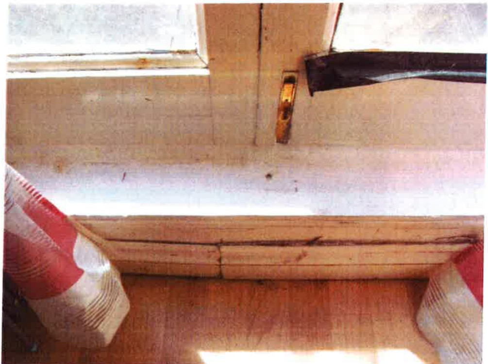
16. Mastic seal/taping at Kitchen door (interior)
