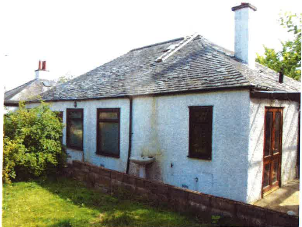
4. Rear elevation showing renewed rhones and downpipes
