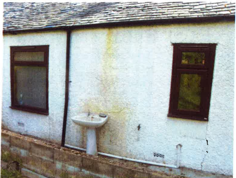
5. Staining to rear elevation from leaking rain water fittings
