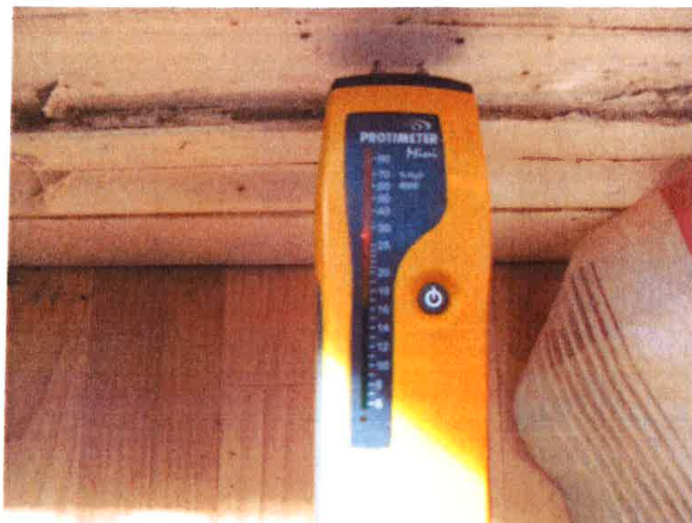
17. High damp meter readings below Kitchen door
