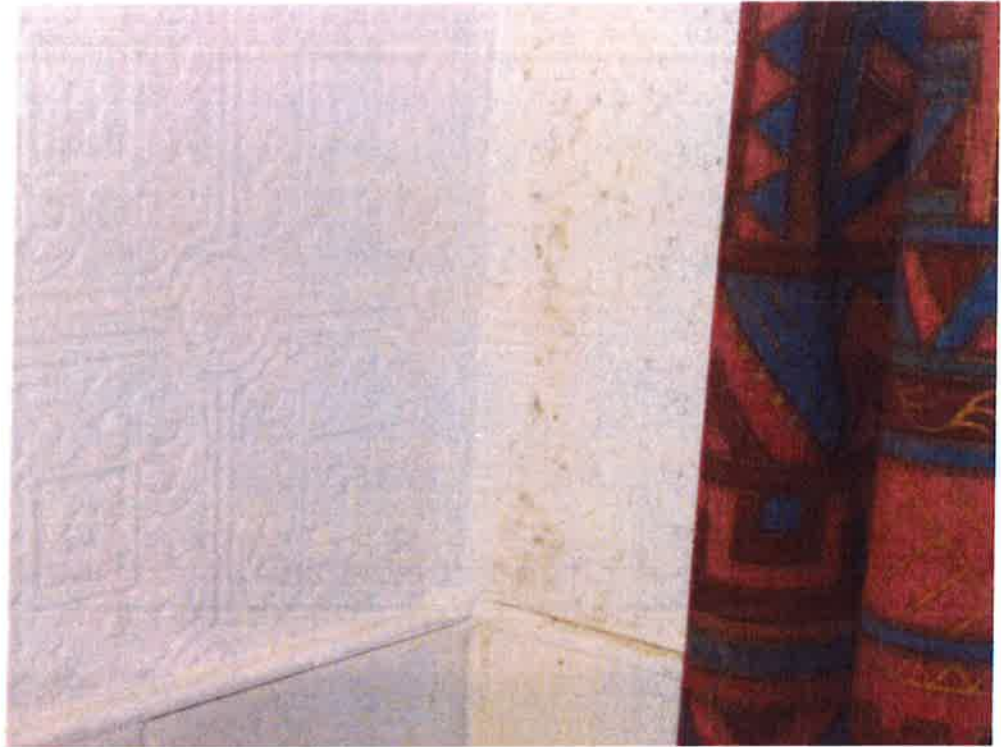
19. Condensation on Bathroom wall
