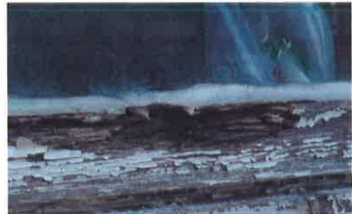
Photo 7 – Rotten kitchen window frame
