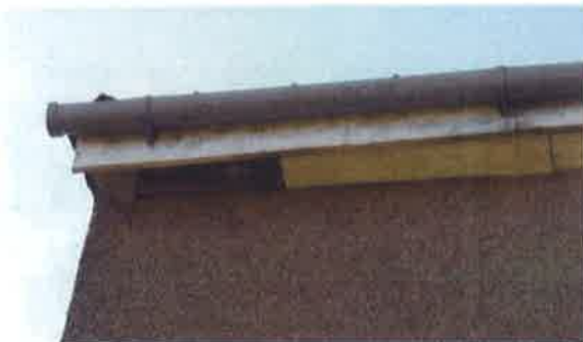
Photo 6 – Missing soffit board
