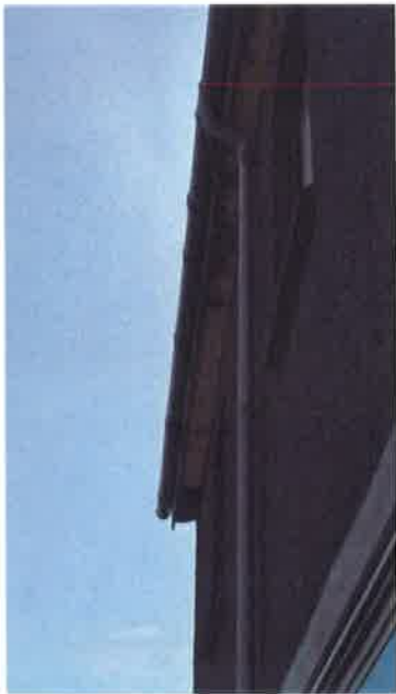
Photo 4 – Soffit and facings – poor order
