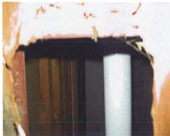
Photo 11 – Exposed flue pipe in bedroom
