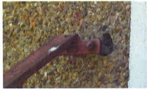
Photo 3 – Insecure handrail
