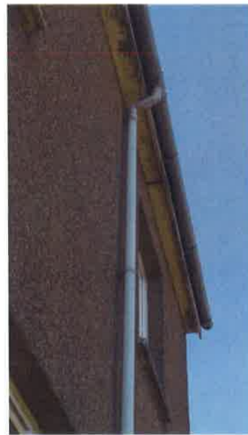
Photo 5 – Soffits and facings - poor order
