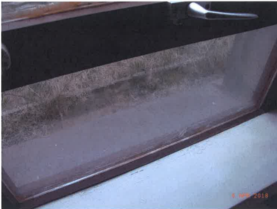
Defective seal to Lounge window (misting between panes of glass)
