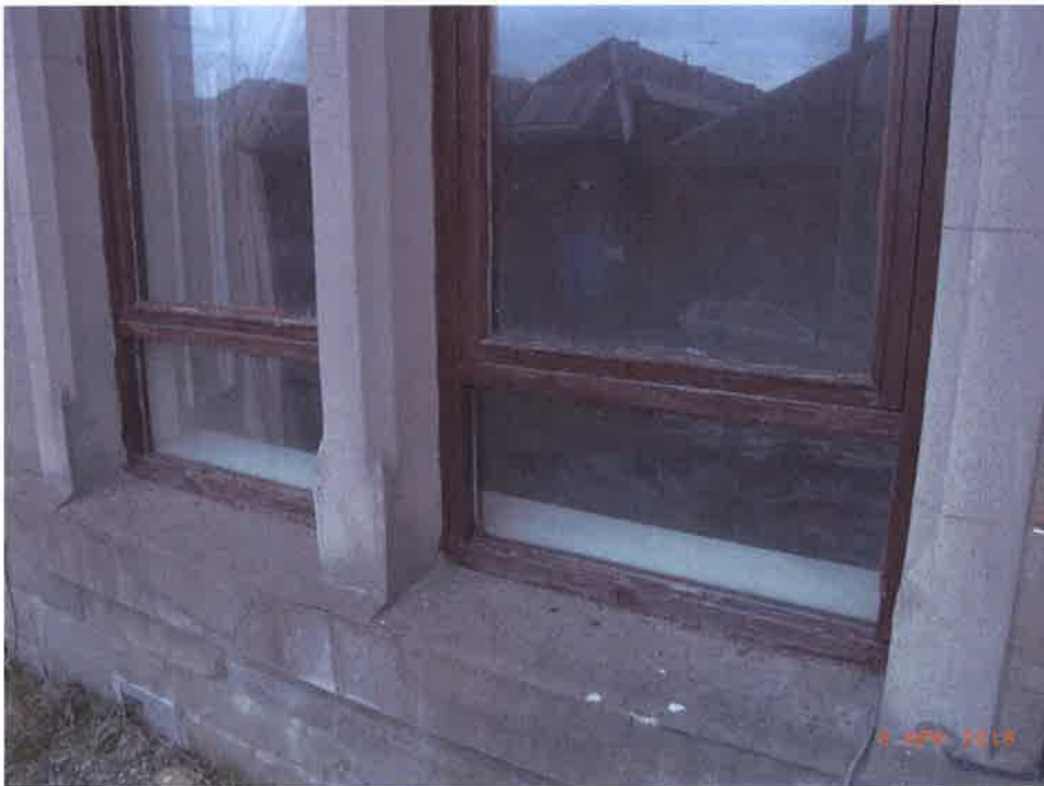
Typical weathering to external woodwork
