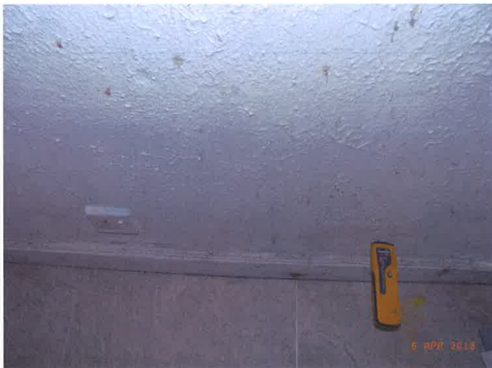
High damp meter readings in close wall of Kitchen
