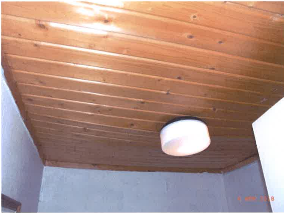
Bow in Bathroom Ceiling
