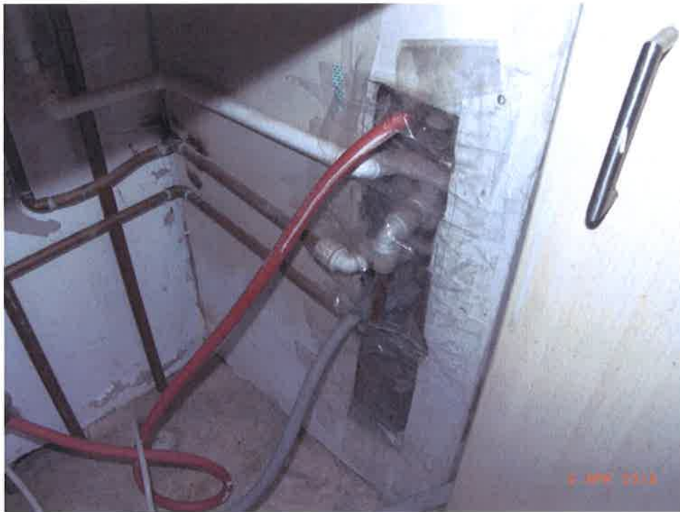
Taped over opening in Kitchen wall lining
