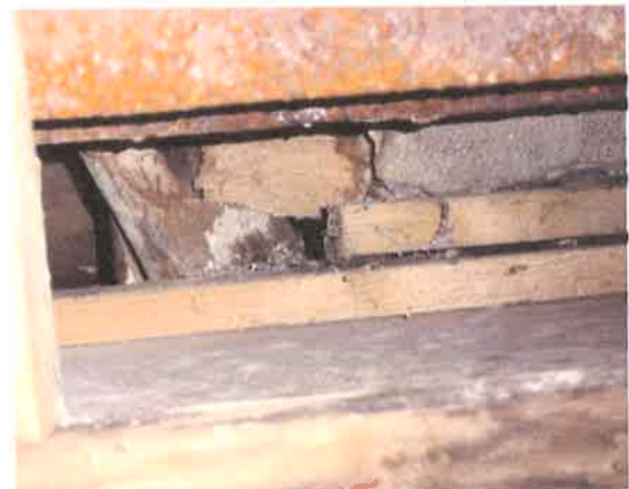
Photographs 8 &9:- Corroded beam & rotted timbers above bedroom window
