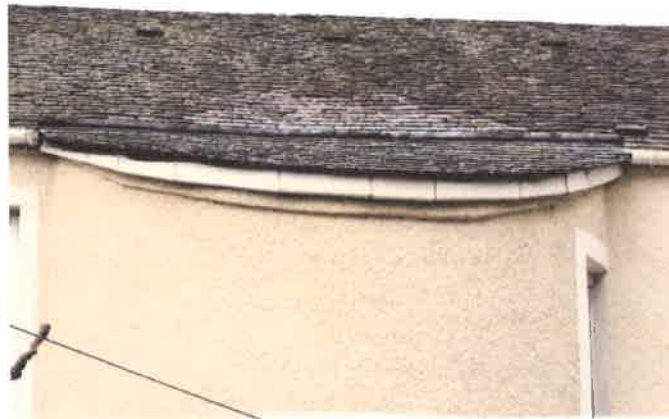
19:- Rain water barrier / diverter above stair projection
