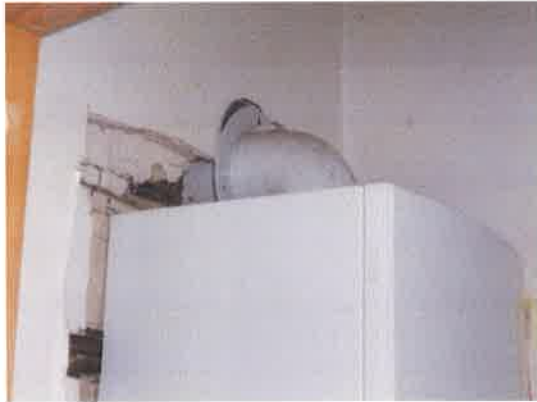
12:- Internal gap at boiler flue
