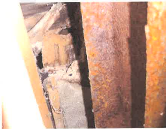
Photographs 8 &9:- Corroded beam & rotted timbers above bedroom window
