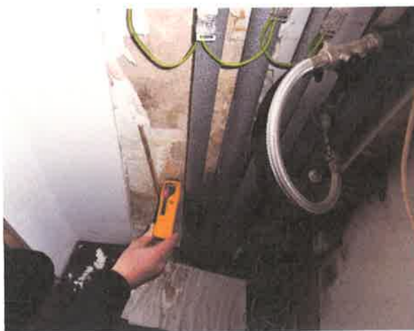
10:- Damp wall below boiler
