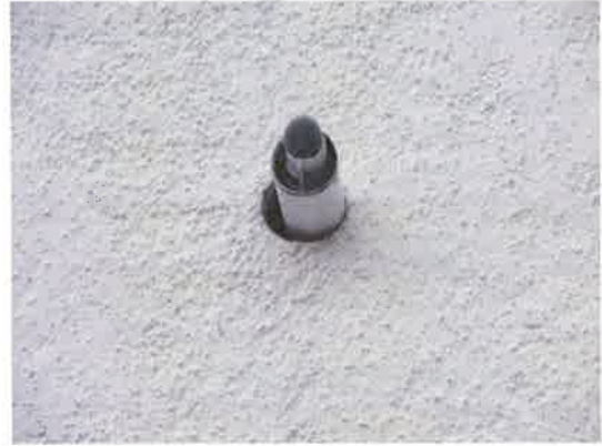
13:- External gap at boiler flue
