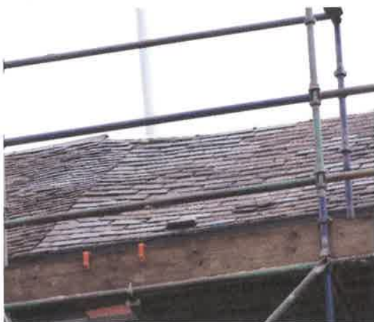
16:- Missing roof slates
