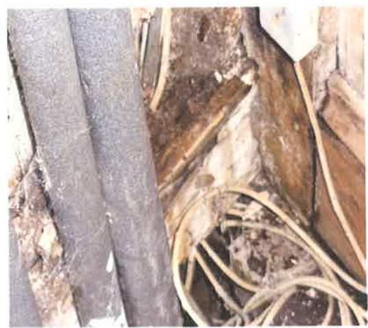
11:- Rotted skirting below boiler
