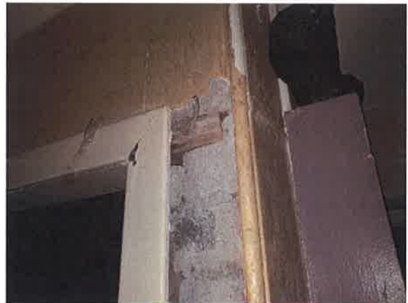
14 Damaged plaster to hall.
