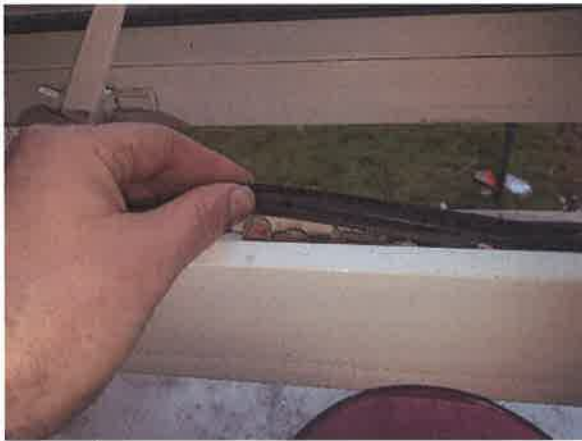
7 Example of loose seal present to window frame.
