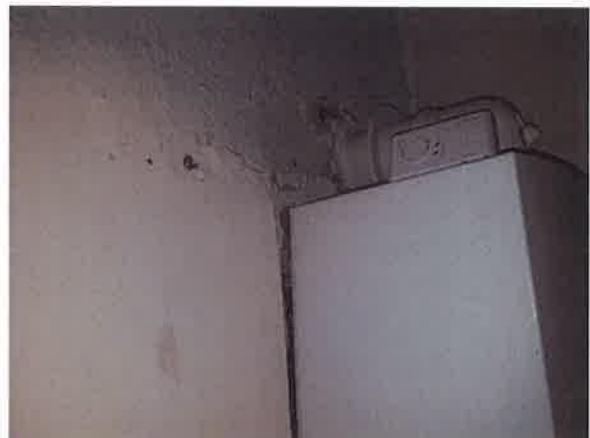
6 Damage to Kitchen walls adjacent to Boiler.
