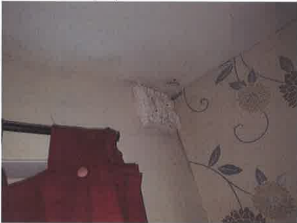
15 Infilled wall vent.
