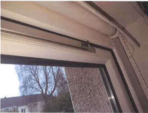
1 Example of trickle ventilation present to windows (except Living Room).
