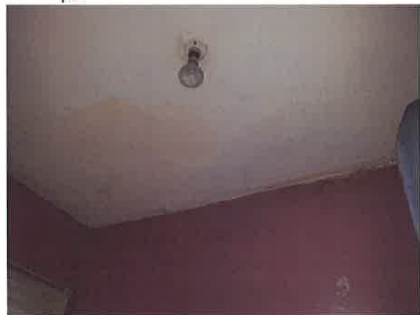
10 Water damage to Bathroom ceiling.
