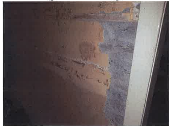
12 Damaged plaster within Hall.
