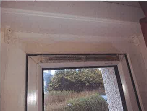
3 Living Room fixed trickle vent – expanding foam present in part.
