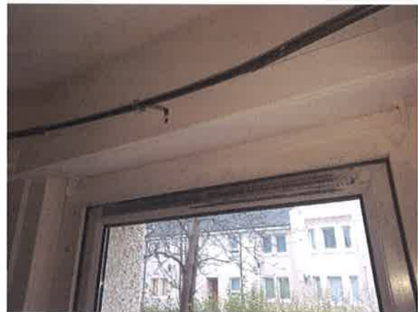
2 Living Room window fixed trickle vent.
