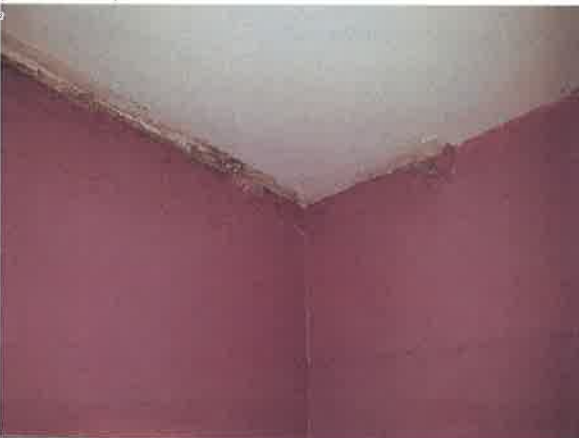
5 View of water damage within Bathroom.
