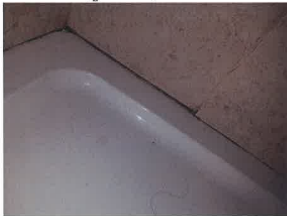
11 Defective seal at shower tray.
