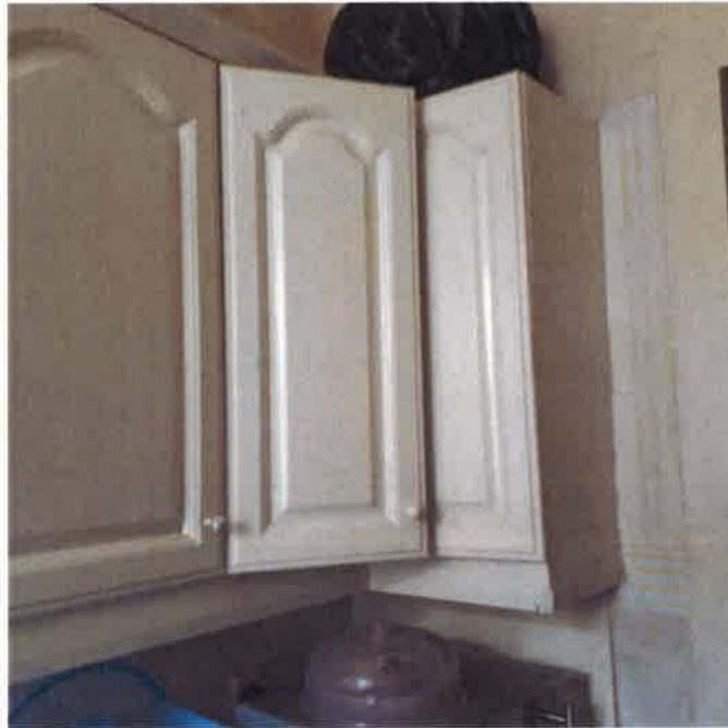
1 Example of ill-fitting kitchen wall unit
