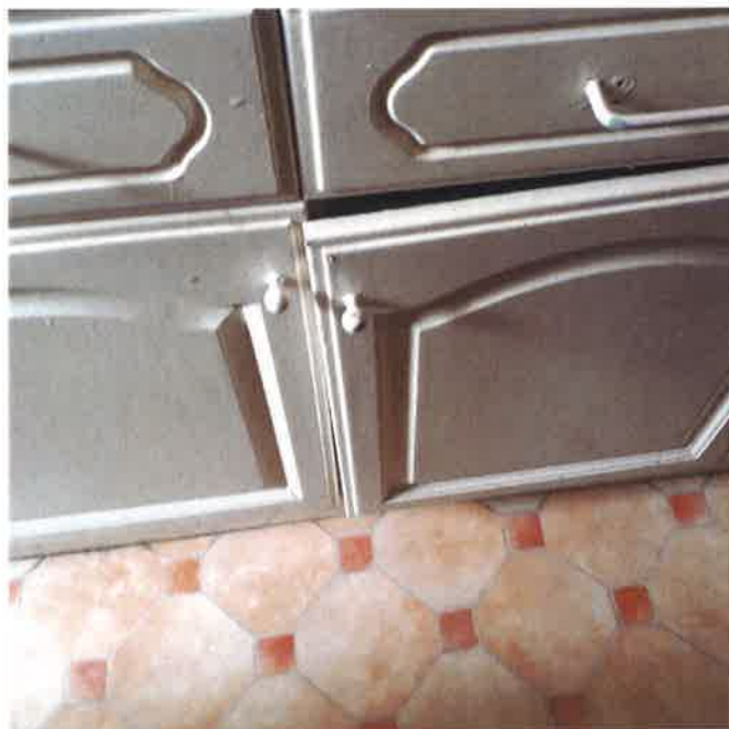
2 Example of ill-fitting kitchen base unit
