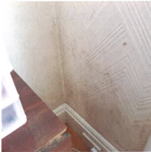
3 Typical example of condensation mould growth at skirting level
