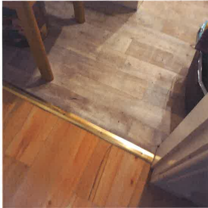
7 The location of the sagging bathroom floor, ripped vinyl flooring and proud nailing
