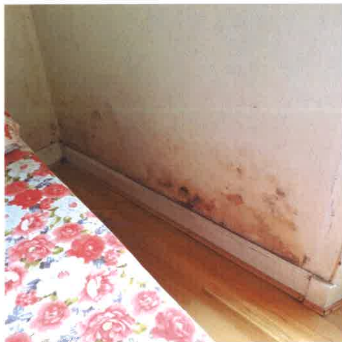
4 Typical example of condensation mould growth at skirting level
