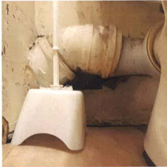
5 The gap in the skirting in the toilet behind the WC
