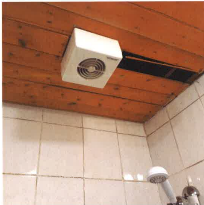
6 Showing one of the missing section of ceiling board in the bathroom
