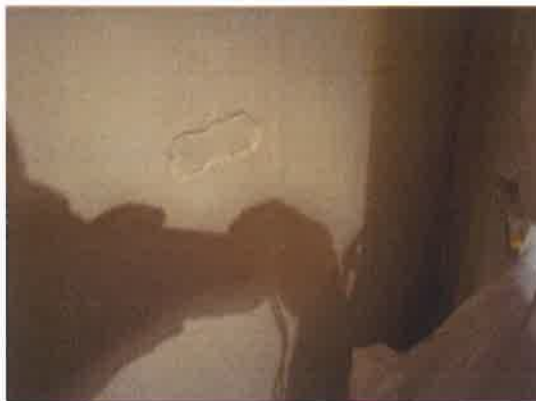
DEFECTIVE PLASTER – KIT WALL
