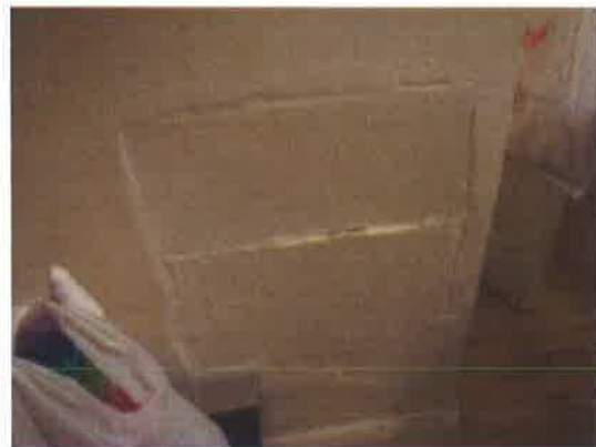
DEFECTIVE PLASTER- KIT WALL
