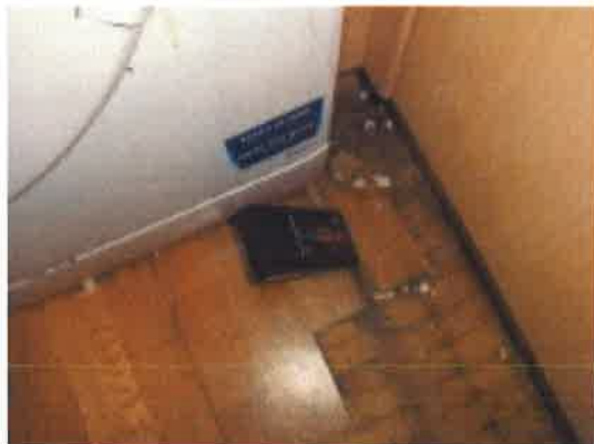
RED “DAMP” METER READINGS AT FLOOR ADJACENT TO WASH MACHINE
