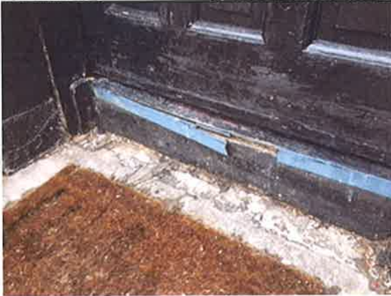
Front Door – Missing Threshold and Weather Bar
