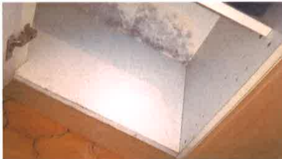
11 Base unit staining to back panel.
