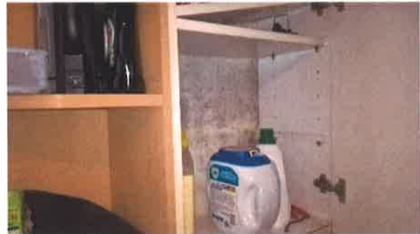
12 Base unit staining to back panel.
