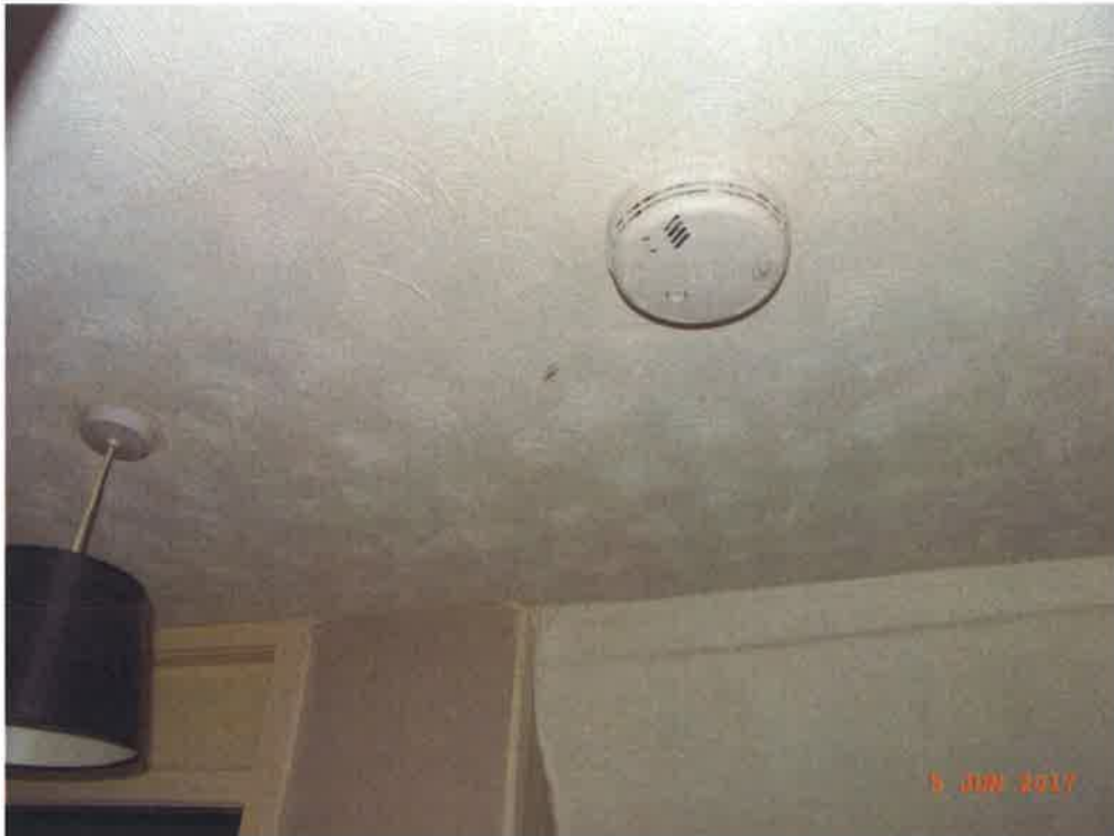
Landing smoke detector
