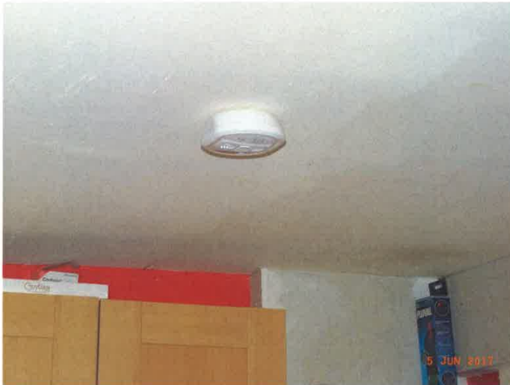
Replacement carbon monoxide detector
