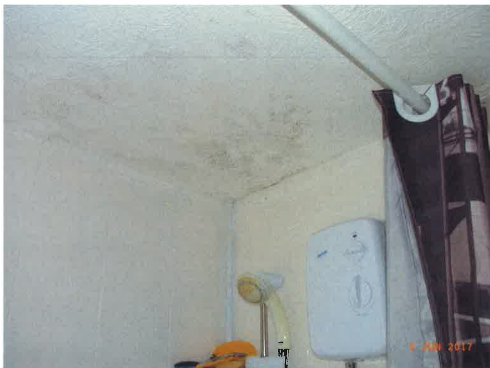
Condensation in bathroom
