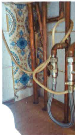
1d)Kitchen: exposed pipes to boiler
