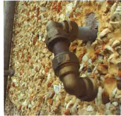
14b Detail of pipe repair
