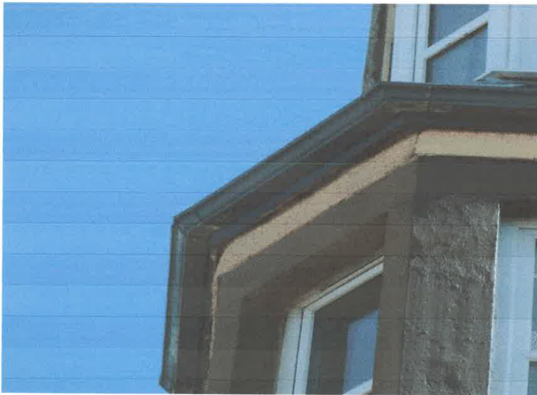
Rainwater goods – one floor above flat. Some refurbishment required, but fascias good
