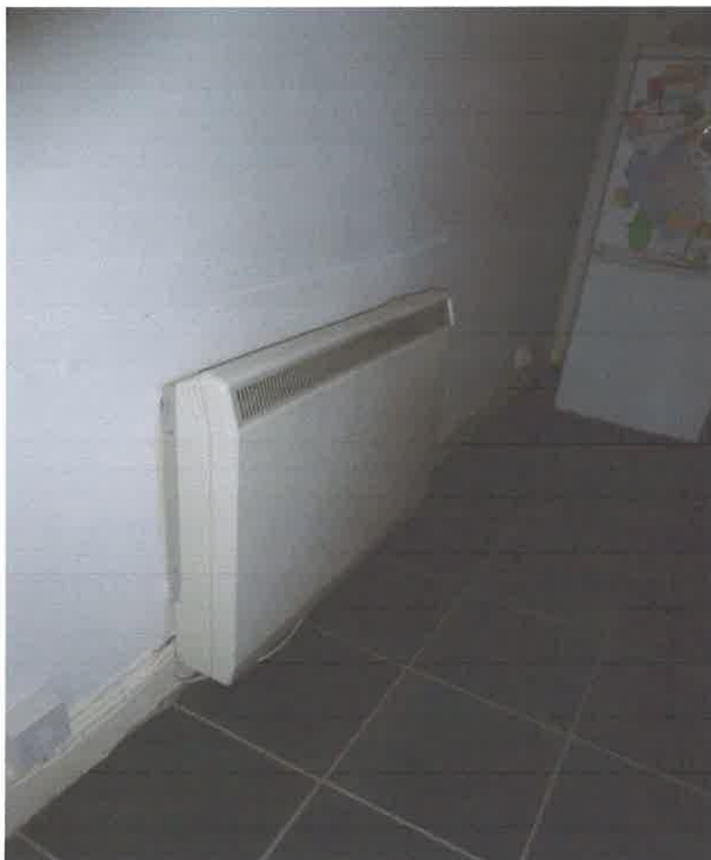
Storage heater to kitchen wall
