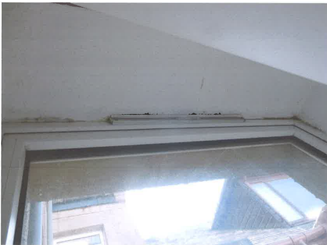
Trickle vents to windows – many closed. Some opened during visit.
