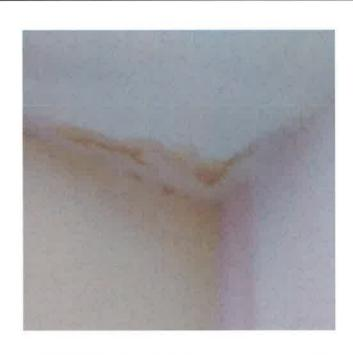
Plasterwork in kitchen wall cracking due to damp
