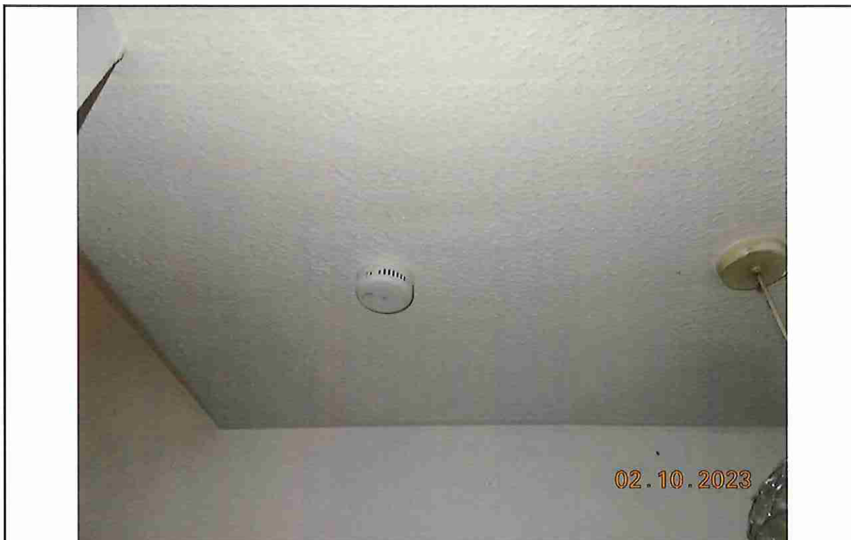
3. Smoke detector and alarm in lower hallway
