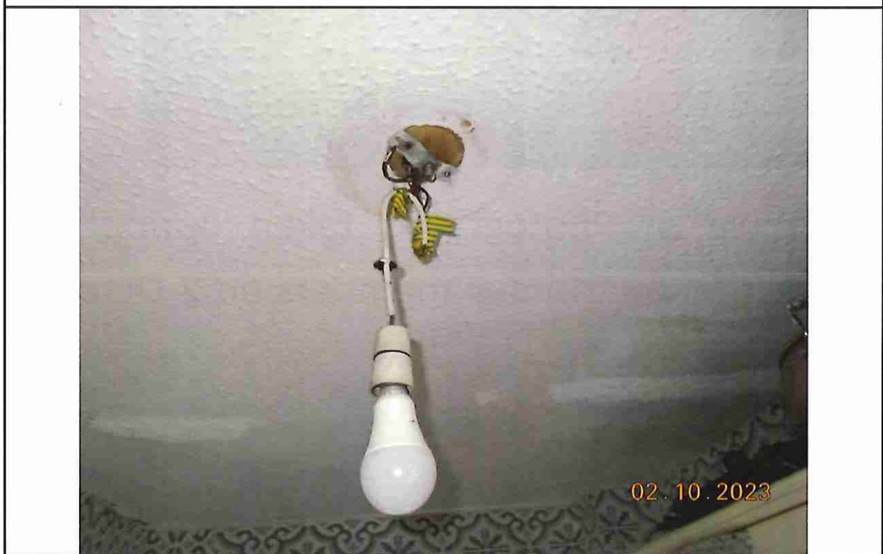
2. Temporary Light Fitting in Kitchen with exposed wiring.
