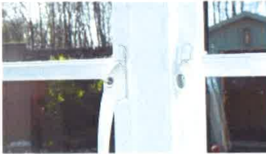
(Ph5) Kitchen window - missing lock
