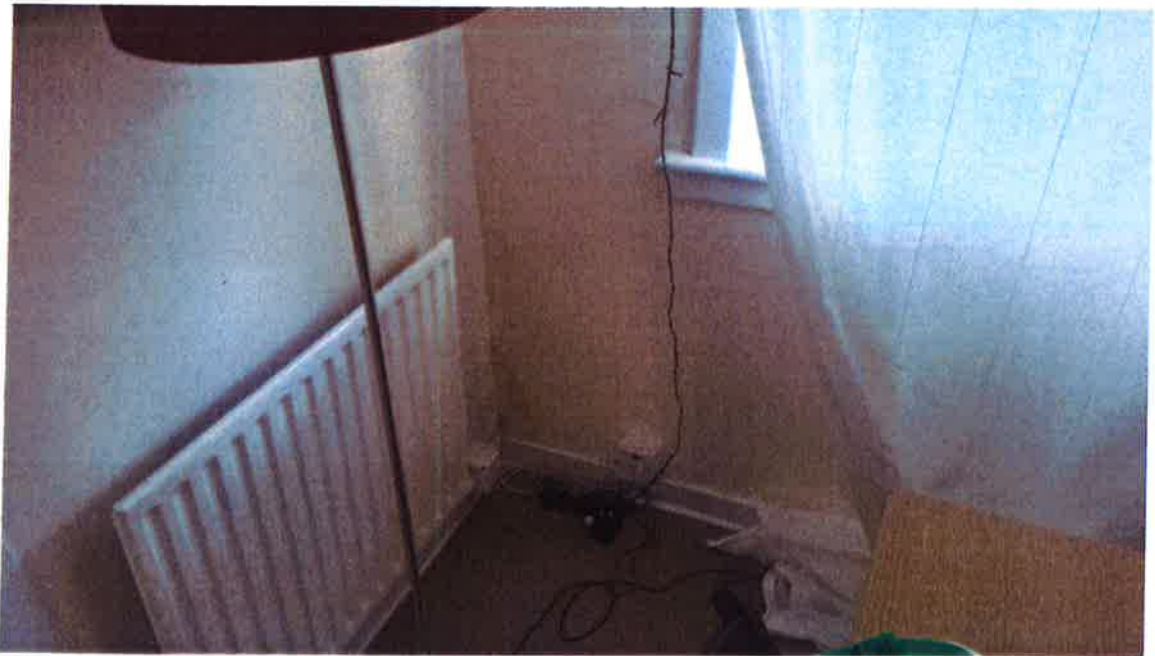
8. Damp staining remains within Living Room below window.
