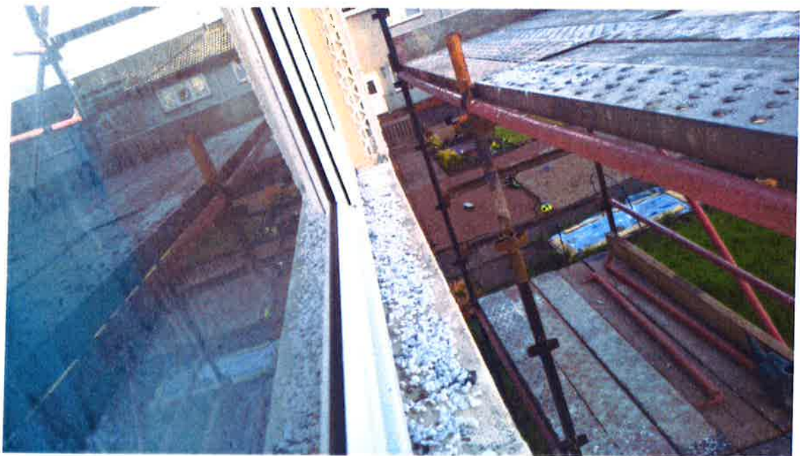
6. View of incomplete rendered jamb at First Floor Bedroom window.
