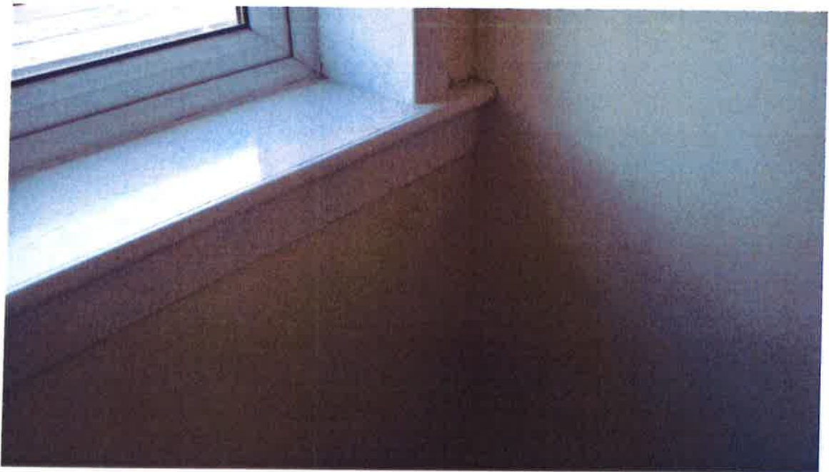
10. First Floor Bedroom – minor damp staining remains.
