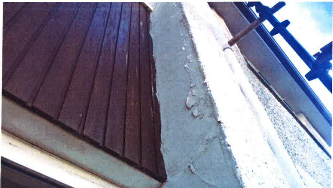
4. Close view of incomplete rendered jamb (right hand side) adjoining timber panelling over Front Elevation.
