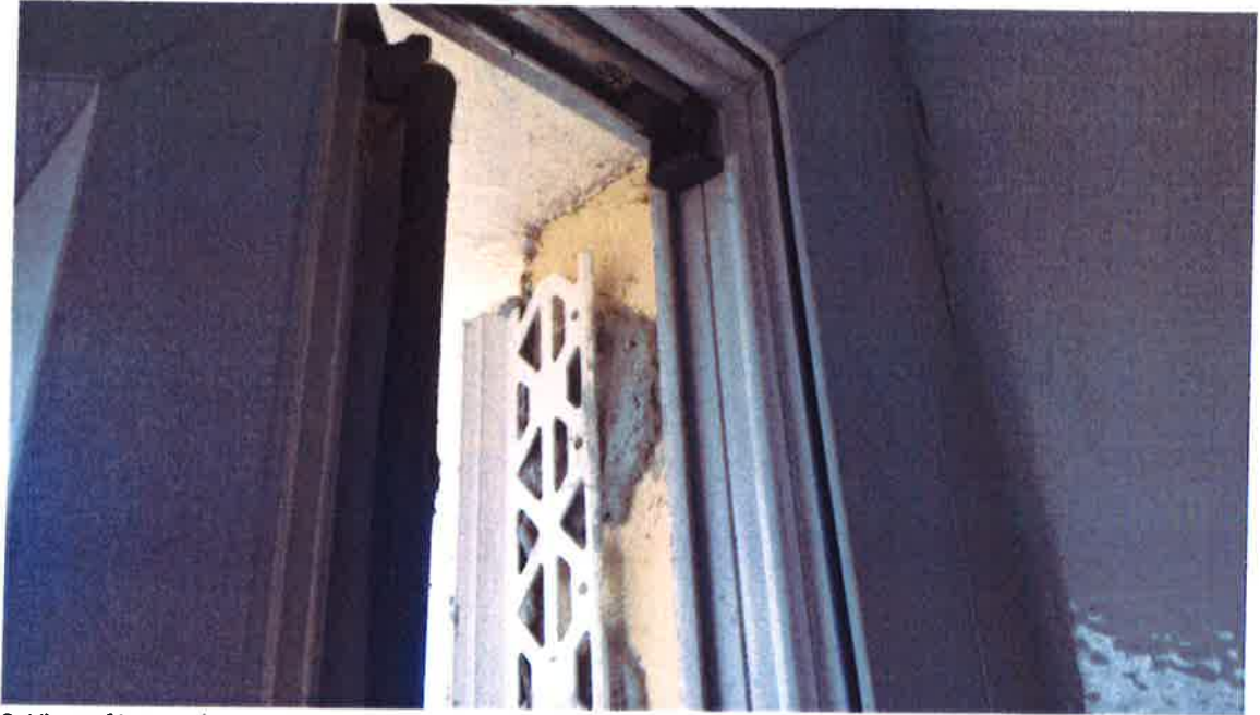
9. View of incomplete rendered jamb.
