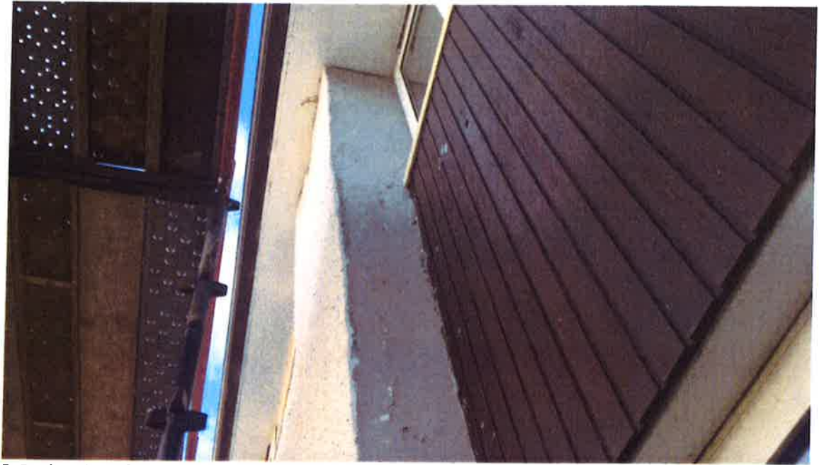
5. Further view of incomplete rendered jamb adjoining timber panelling (left hand side)
