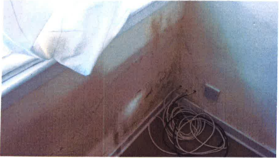
7. Damp staining remains within Living Room below window.
