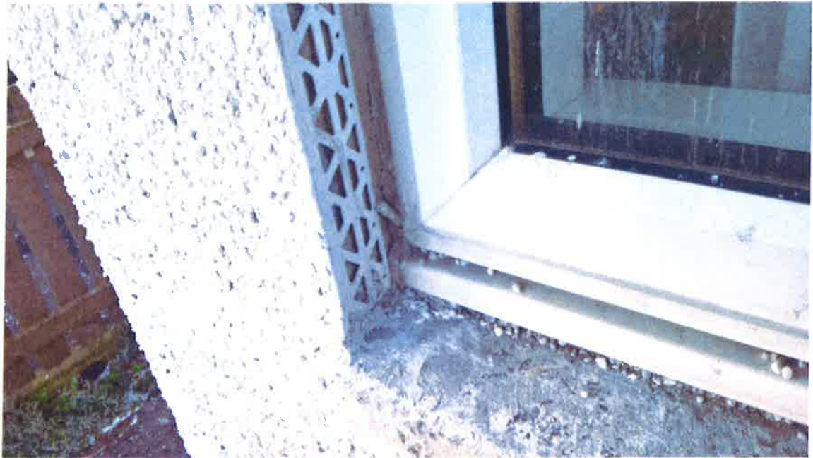
3. Close view of Front Elevation ingoe/jamb of Living Room window – render incomplete.
