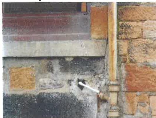
Rear Wall 13 January 2020
