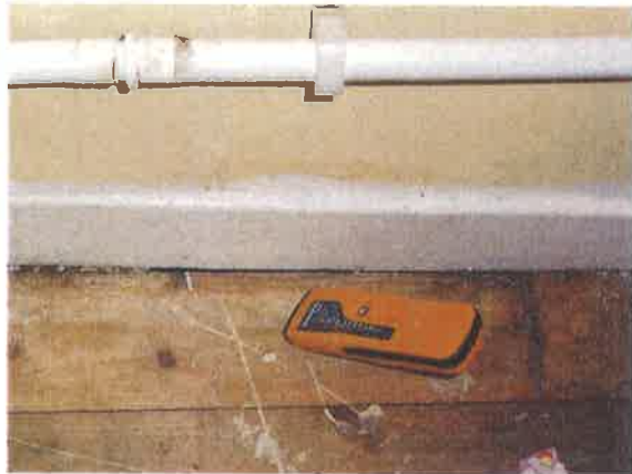
Repaired condensate pipe 13 Jan 2020
