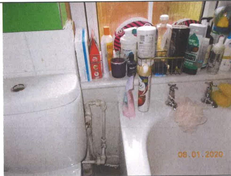
4. Filled hole in external wall to the Bathroom
