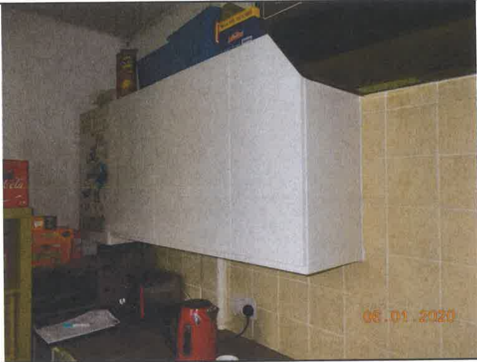
3. Replaced Kitchen wall units
