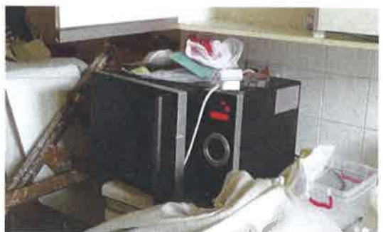
Photo 5 – Portable appliance in kitchen
