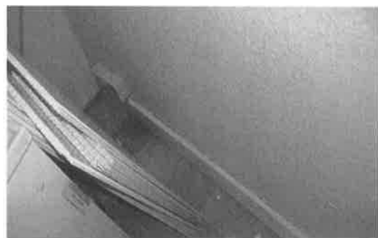
Photo 3 – New skirting in kitchen
