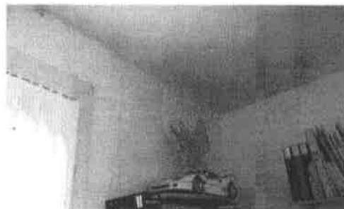
Photo 5 – Repaired wall at 14/11/19
