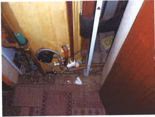
14. Floor of boiler cupboard
