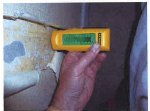
13. Damp meter check bedroom wall
