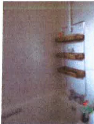
Bathroom - new wet wall panelling
