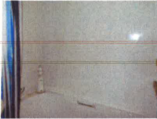
Bathroom - bath and bath panel sealed properly
