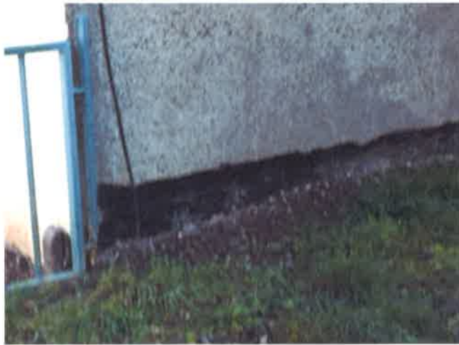
Side elevation - showing works carried out by builder
