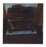
Gas fire with back boiler. No Gas Safe Certificate and no Carbon Monoxide detector.
