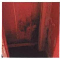
Dampness and mould in bedroom cupboard on east external wall
