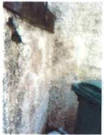
Steps to entrance to first floor flat No 7A(East elevation). Junction of steps with main external wall would correspond approximately with dampness in main bedroom cupboard.
