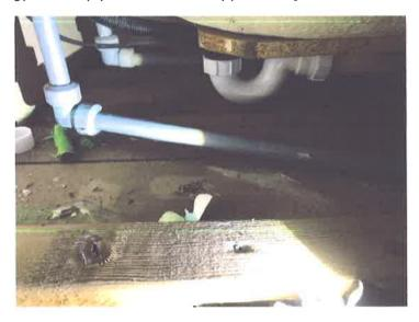
h) No repairs to sealant around bath. Bath was full of water as unable to drain away due to blockage in pipe.
